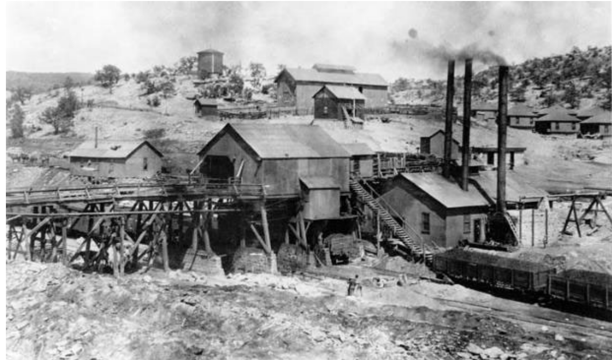
Weaver Coal mine, Gallup, NM. From NMBGMR photo archive.
