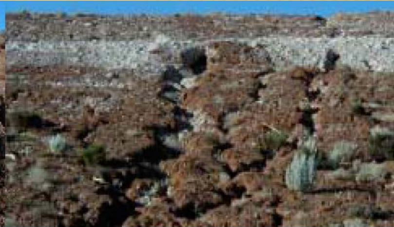
Tunnelling through a berm
