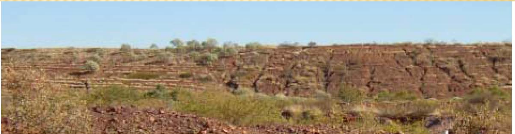
Waste dump with small rip lines and little erosion on left, large rip lines and gullies on right.
