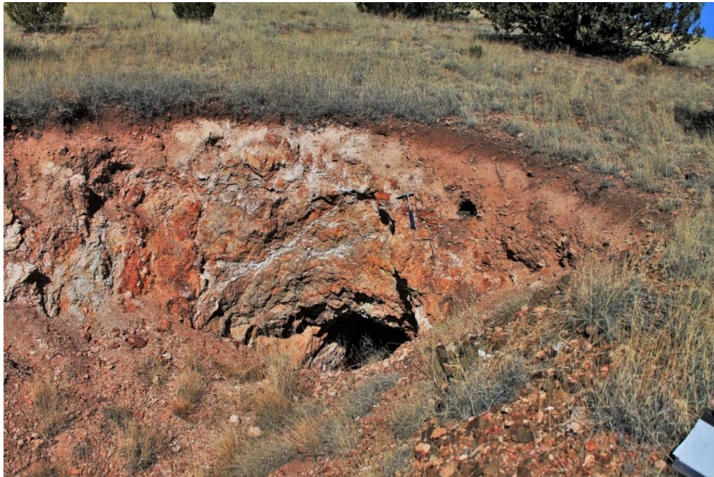
Figure 14. NM354-A1 (NMSO0879); an untimbered adit in extremely altered rock.
