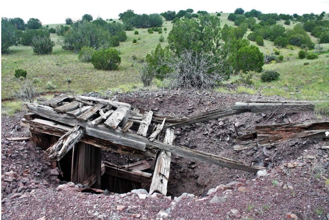
Figure 12. Mag4-S1 (NMSO0377); main shaft on the Chief vein sank ca. 1919 (Lasky, 1932). Headframe collapsing into collar of shaft (¼ mi from NM-169).
