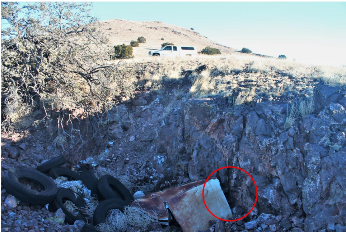
Figure 15. SH-S2 (NMSO0898); deep shaft plugged with trash. Circled area is opening to shaft below. Note proximity to road above.
