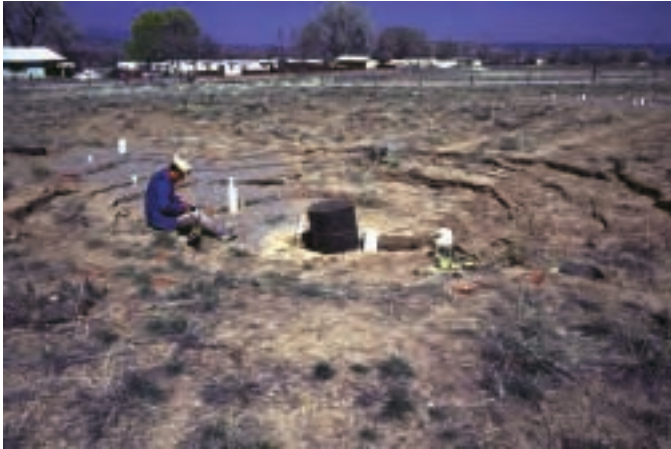
FIGURE 1—Ground subsidence of 2.2 ft affecting an area of 600 ft 2 after injecting nearly 17,000 gallons of water into the soil at a depth of 10 ft over 16 days (water equivalent to septic tank use by a family of four for 1 month). Collapse was initiated within 1 week.
