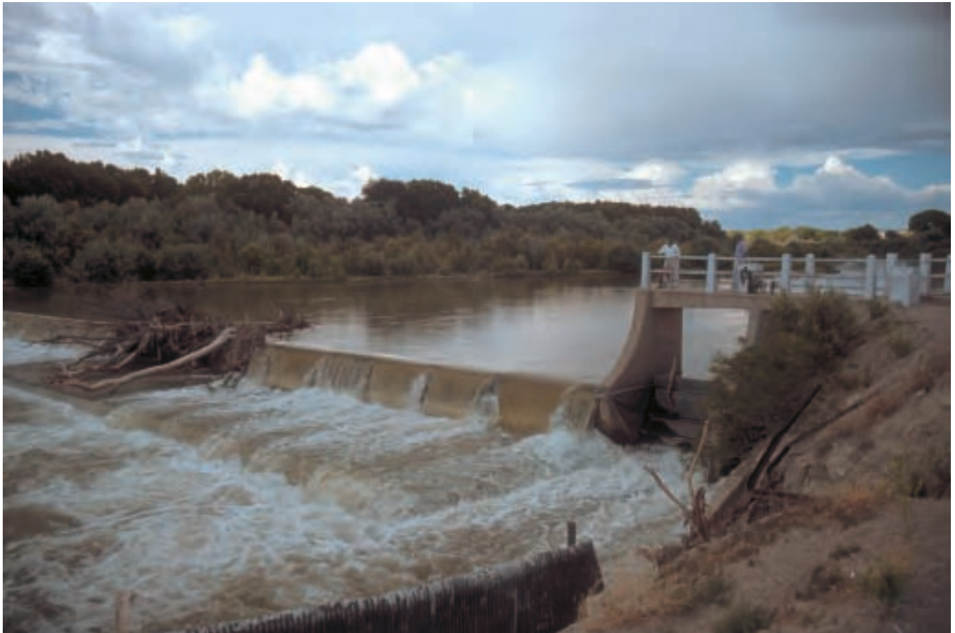
The Angostura diversion dam, operated by the Middle Rio Grande Conservancy District, is one of three major diversions of irrigation water along the middle Rio Grande valley. The dam was constructed in 1934 and rehabilitated by the Bureau of Reclamation in 1958. It has the capacity to divert 650 cfs to the Albuquerque Main Canal. It consists of a 800-ft-long concrete weir that has a structural height of 17 ft and a hydraulic height of 4.5 ft. Photo by Paul Bauer, August 2000.
