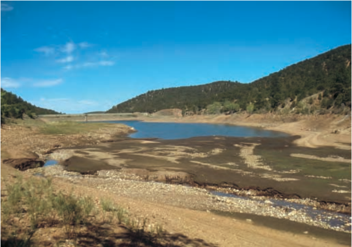
View downstream of McClure Reservoir on the Santa Fe River during the dry summer of 2000. The reservoir level is low enough to reveal the sediment delta (dark-colored flat area in lower half of photo) that the river built up during wetter years. Over time, the accumulation of such sediment decreases the storage capacity of the reservoir. Note that the Santa Fe River is reduced to a trickle (lower right), and it has eroded a channel into the sediment delta. Photograph by Paul Bauer, August 2000.
