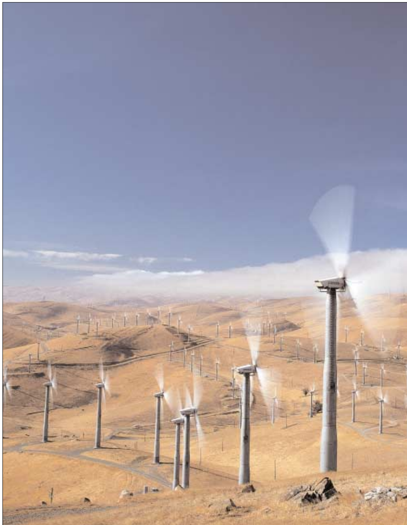
Wind turbines at Altamont Pass, California
