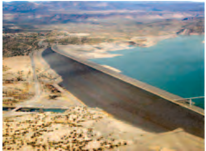
Cochiti Dam and Reservoir
