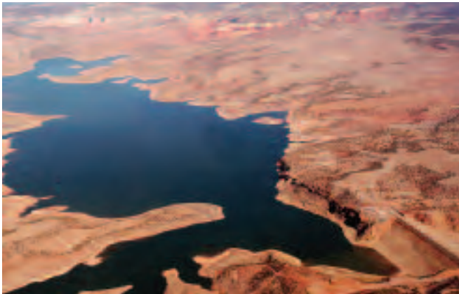
Abiquiu Dam and Reservoir
