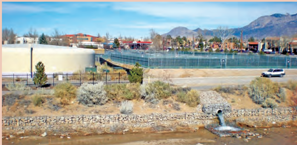
The Bear Canyon Recharge Demonstration Project on Bear Canyon Arroyo, approximately seven miles from the Rio Grande. Water is pumped from the river to the storage reservoir (visible on the left) and is then discharged into Bear Canyon Arroyo, where it seeps into the subsurface within a mile of the reservoir, thus recharging the local aquifer.
