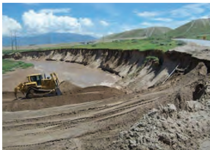
Repairing bank erosion along Tijeras Arroyo in 2006.
