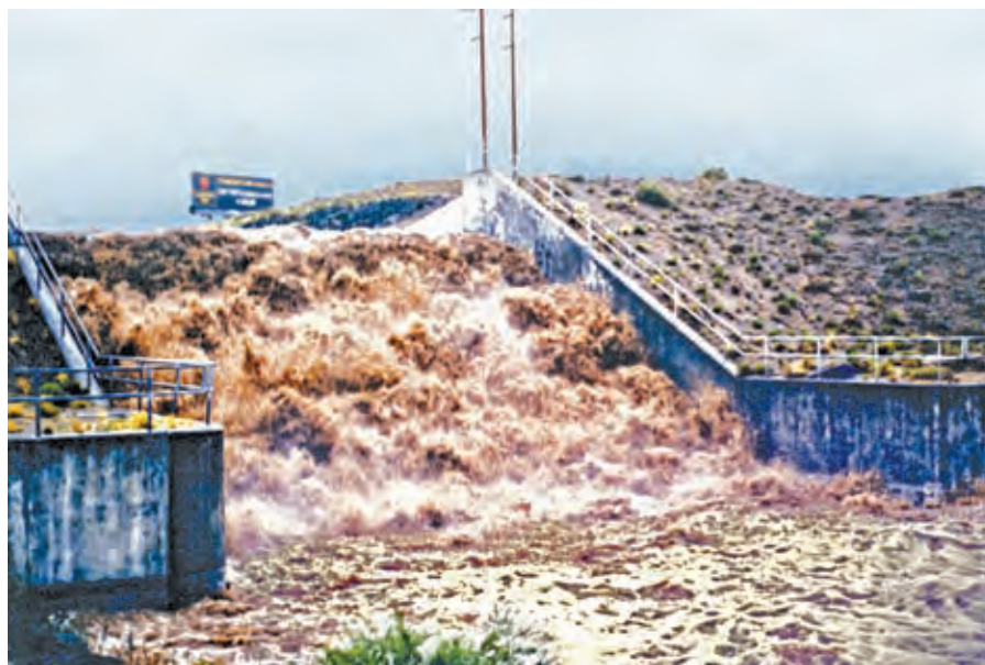
Floodwaters during the July 14, 1990 flood, AMAFCA South Diversion Channel baffle chute, just west of I-25, the highest flow on record at 2,300 cfs.
