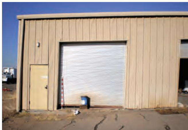
Buckling of the south end of the Kaibab Warehouse #1 at the city's Montessa Park facility due to soil collapse of about 2.5 feet. The cracks in the foreground encircle the deepest part of the collapse feature, to the left of the building. Runoff from the roofs, pavement, and facility water use entered the soil, causing it to compact. Subsurface tests show that more subsidence is likely unless all surface runoff is eliminated.
