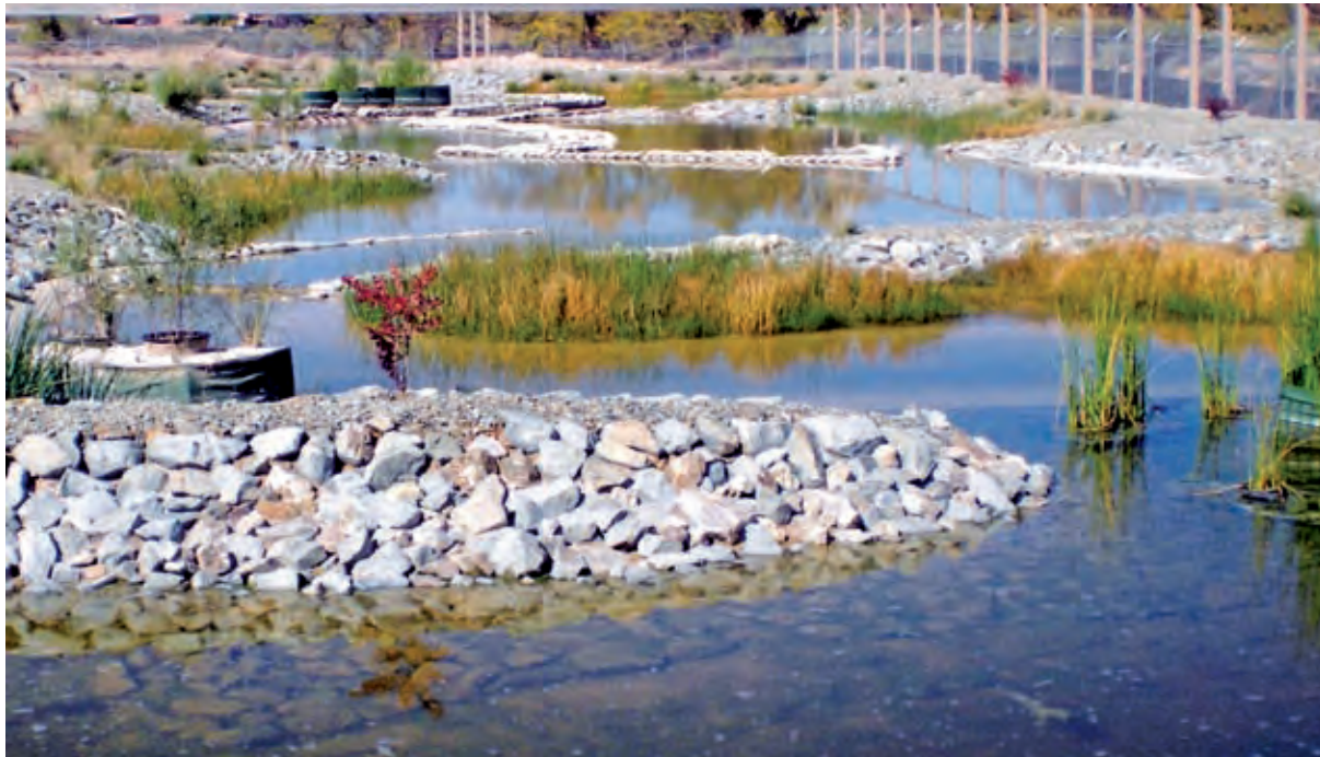
The Los Lunas silvery minnow refugium, a project of the New Mexico Interstate Stream Commission. The refugium provides a 460-foot-long meandering stream with ponds and overbank features that function like natural environments in the Rio Grande.
