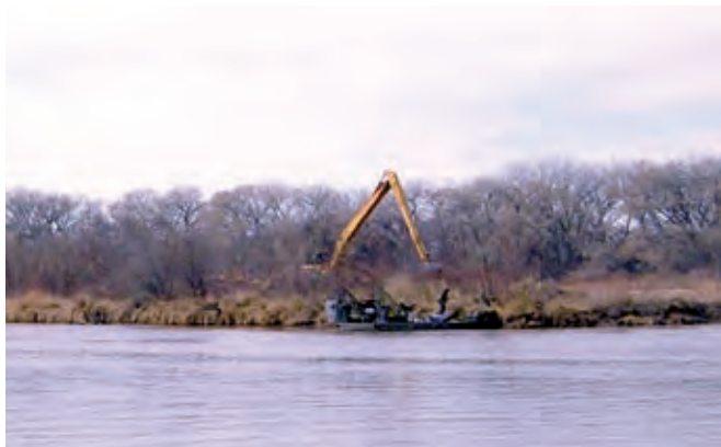
Left: Amphibious earthmoving equipment removing and redistributing sediment from a high-elevation, mid-channel island in the Rio Grande south of Albuquerque during construction of floodplain habitats subject to inundation at lower magnitude spring flows (3,000 cfs); winter 2006. Right: The same island nine months later, showing regrowth of vegetation and establishment of new wetland vegetation that promotes egg retention and provides excellent habitat when flooded for silvery minnow rearing; fall 2006.
