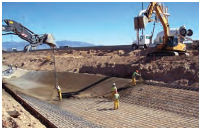
Building the lining for the Amole Arroyo on the west side of the Rio Grande, using tinted shotcrete.
