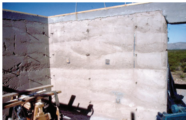
Figure 5. Rammed earth walls topped by concrete bond beams. Photo by George S. Austin.
