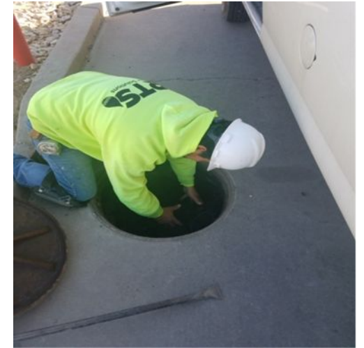
Water Meter Retro Installation
