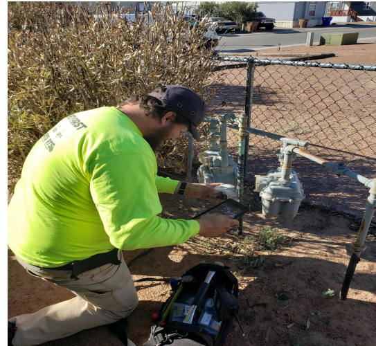
Gas Meter Retro Installation
