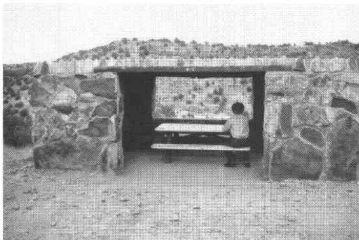
FIGURE 5—Rock shelters made of Yeso sandstone along the upper loop, view looking across the Pecos Valley.
