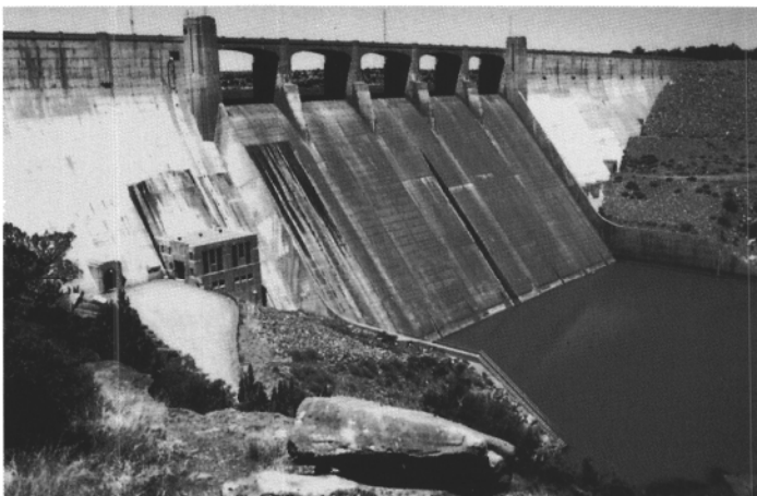
FIGURE 2—Conchas Dam, looking northeast.
