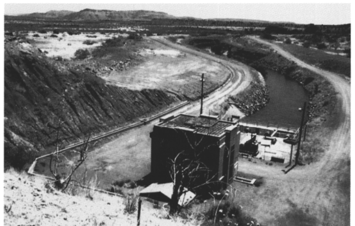
FIGURE 3—Headworks of the irrigation system.
