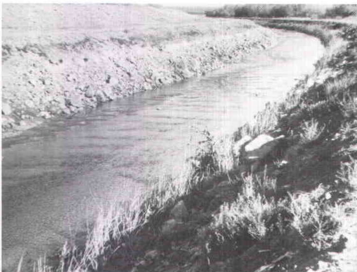
FIGURE 2—Low flow in conveyance channel of Rio Grande near Socorro on April 19, 1984. Note tops of megaripples near water surface. Channel is approximately 10 m wide.
