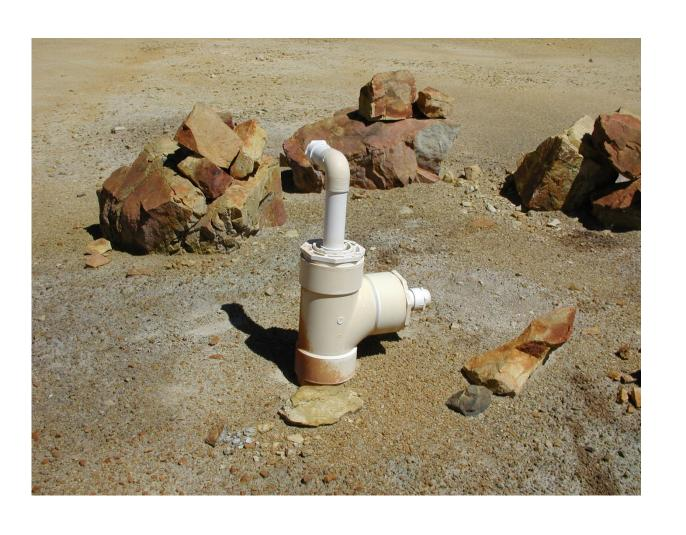
Monitoring wells are throughout the mine area to measure differences in water levels, chemistry, and water flow. Hydrologists use these data to model and predict the water flow and quality before, during, and after mining.
