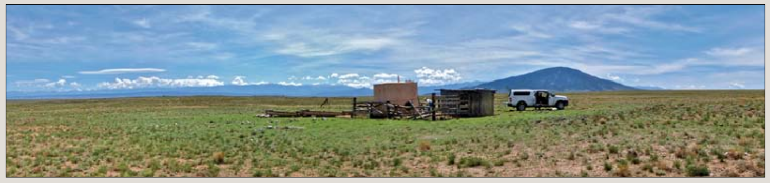
Taos Plateau water well and tank, with Ute Mountain in the distance.
