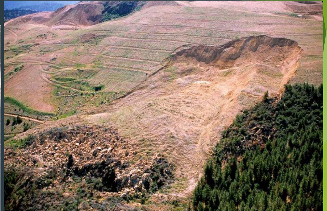
Hayden Hill Gold Mine Waste Rock Failure, Copyright AMEC
