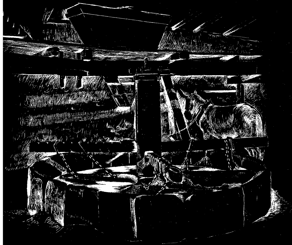
THE ARRASTRA: ONE OF THE MOST FAMOUS TECHNICAL DEVICES UTILIZED BY MINERS IN NEW MEXICO DURING THE SPANISH PERIOD AND MOST OF THE 19TH CENTURY. THE ARRASTRA WAS USED TO GRIND AND AMALGAMATE GROUND MILLING GOLD AND SILVER ORES OR TO GRIND VARIOUS ORES FOR REDUCTION IN FURNACES.
