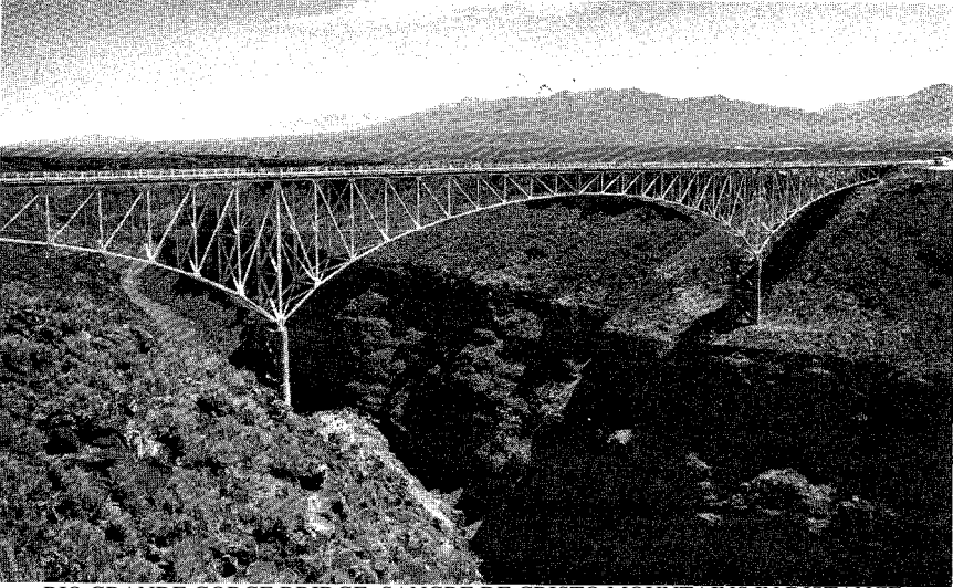
RIO GRANDE GORGE BRIDGE; SANGRE DE CRISTO MOUNTAINS IN DISTANCE.
