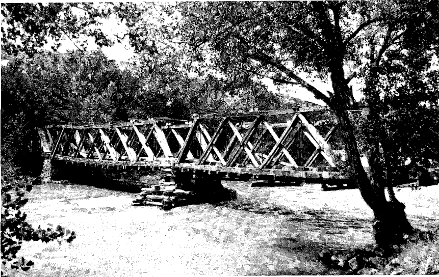
OLD EMBUDO BRIDGE ACROSS RIO GRANDE; mile 27.8, Taos-Española log.
