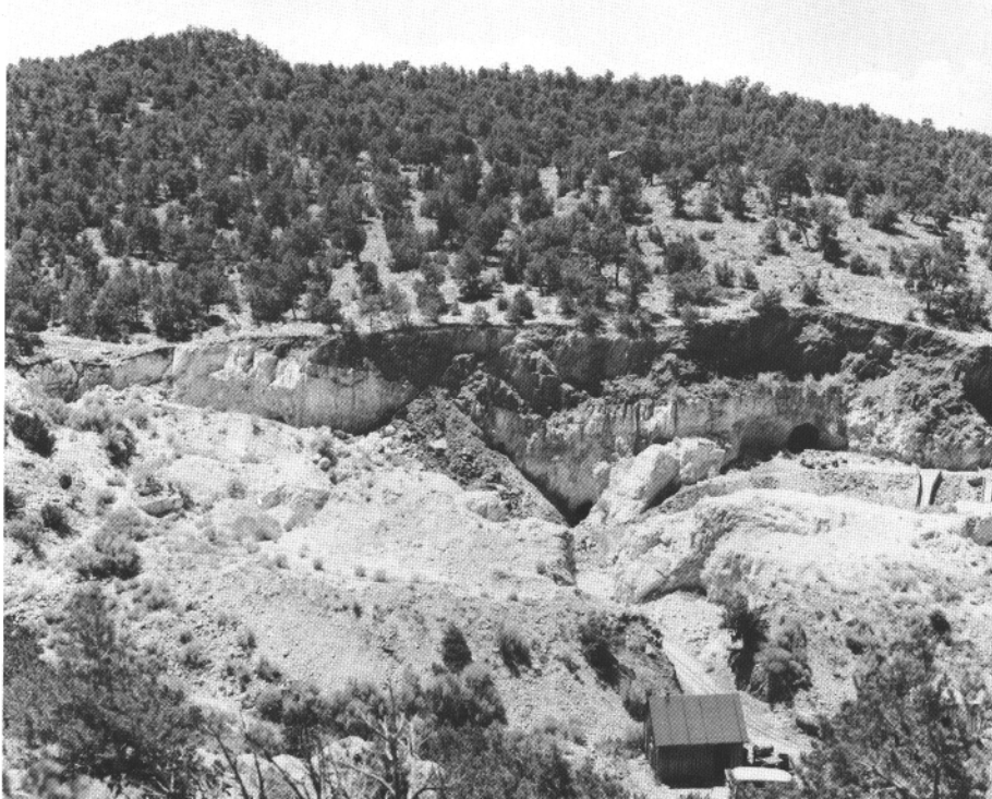
Southwest view in 1953 of the main quarry of the Harding pegmatite mine from North Knob. The upper contact of the pegmatite with the darker Precambrian metamorphic country rock can be easily identified. Three underground entrances to the mine are visible. The lowest tunnel at the end of the road is the entrance to the large lepidolite room. To the left and upslope is the entrance to the microlite tunnel, and upslope to the right is the tunnel to the beryl workings. If you have a keen eye you'll see five men sorting beryl at the tunnel entrance. Ore also was dumped down the wooden chutes for sorting. The buildings in the foreground are mine buildings; the building on the wooded slope behind the mine is a temporary structure of the U.S. Bureau of Mines. © 1981 Laura Gilpin Collection, Amon Carter Museum, Fort Worth, Texas.
