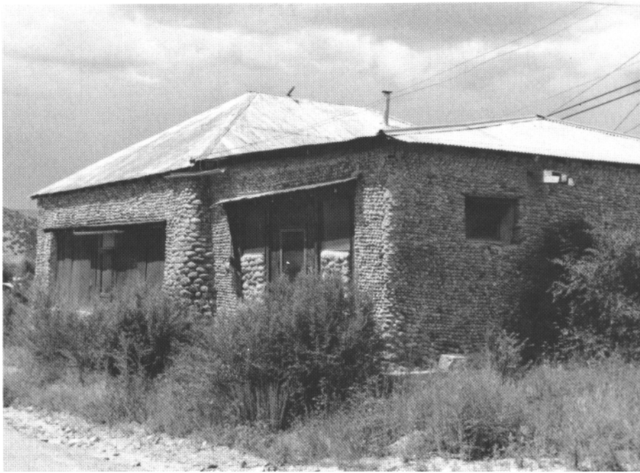
Old Dixon store constructed of river-rounded quartzite boulders of the Precambrian Ortega Formation. Corrugated galvanized steel roofing is common in rural northern New Mexico.
