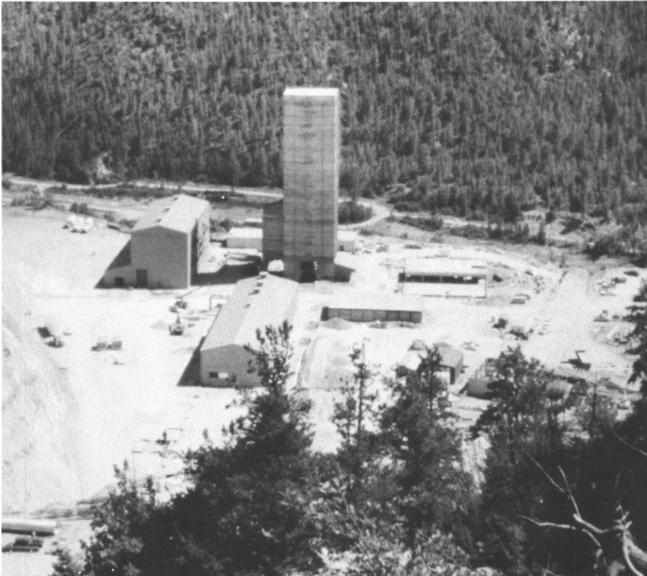
Headframe of Molycorp mine's service shaft for the new underground workings near Goat Hill. Photo courtesy of Molycorp, Inc.
