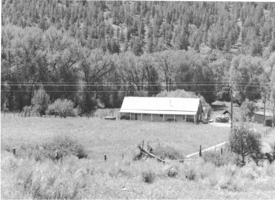
Rural home in the Rio Pueblo valley illustrates the traditional Spanish Colonial floor plan with rooms in a single line. Near 7,700 feet in elevation, the pitched metal roof becomes important for shedding rain and snow.
