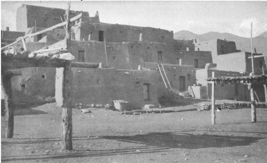
North pueblo, circa 1905. Taos Pueblo is the only large, multi-storied pueblo remaining today. The north pueblo has five levels. Originally, for protection from nomadic Indian raids, the lower level was constructed without doors, and entry was gained by climbing a ladder and entering through a hole in the roof. Photo by B. G. Randall, courtesy of Las Quince Letras.
