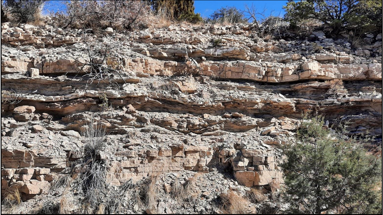
Figure 5. A roadcut exposure of the Queen Formation showing thin- to thick-bedded light-orange sandstone. The thicker, lighter-colored layer near the top is dolomite. This location is along the Guadalupe Ridge Road at Klondike Gap.
