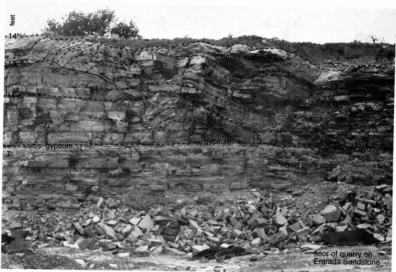
FIGURE 10—Billy the Kid mine section 88J-3, studied on the extensive highwalls of an active quarry. The Todilto Limestone Member section is 14–15 ft (4.3–4.6 m) thick. The quarry floor is on the top of the Entrada Sandstone, and the limestone is overlain by maroon sandstones of the Beclabito Member, Wanakah Formation. The lower platy zone is 7 ft (2.1 m) thick and is composed of angular grains of detrital quartz floating in a matrix of neomorphic microspar calcite. This zone is capped by a 1–2 inch (2.5–5 cm) bed of white gypsum followed by the middle crinkly zone, 8.7–9.7 ft (2.7–3.0 m) of arenaceous ostracode–lime mudstone. The massive unit is 1 ft (0.3 m) of arenaceous ostracode–lime mudstone. The contact with the overlying Beclabito Member sandstones is gradational over a thickness of 1–2 ft (0.3–0.6 m). Small intraformational folds are developed at the base of the middle crinkly zone and extend to the top of the section.
