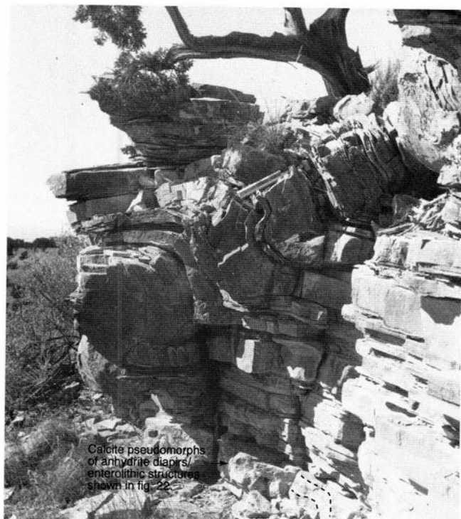
FIGURE 31—A natural exposure of an intraformational fold developed in the middle crinkly zone in the Zia/La Jara area. The north half of the fold is preserved on a cliff. The fold is underlain by supratidal sediments that have calcite pseudomorphs of gypsum/anhydrite mush and anhydrite diapirs/enterolithic structures. A 6 inch (15 cm) scale is shown in upper center of photo. See Figure 22 for photos of these sedimentary structures.
