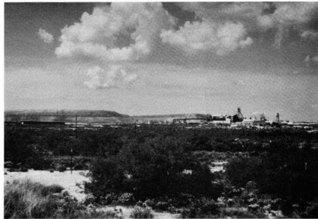
FIGURE 6—View, looking south, of the Eddy Potash (former PCA) mine and mill showing large tailings piles composed mainly of salt with lesser amounts of clay-size particles (slimes) and minor hematite.
