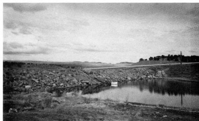
FIGURE 8—Dam-facing made of large clinker material at Peabody Black Mesa mines, northeast Arizona.
