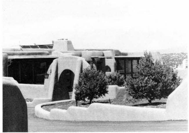
FIGURE 81—Large pressed-earth-block home built with Ridge Adobe pressed-earth blocks made by the Goldbrick "5000" machine, La Tierra area near Santa Fe.
