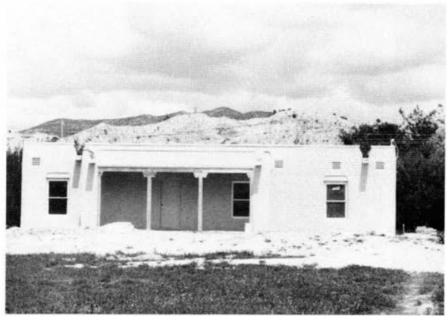
FIGURE 85—Completed HUD pressed-earth-block house built with the Goldbrick "5000" machine, Nambé Pueblo.
