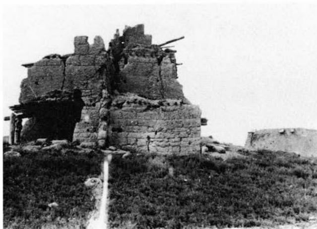
FIGURE 6—Puddled Adobe Structure at old Picuris Pueblo, ca 1900. Note size of puddled adobes that were patted into place by hand. Photo by A. C. Broman.
