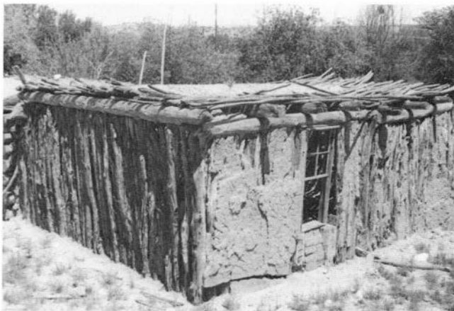
FIGURE 3—Old house near Abiquiu. Jacal construction using cedar poles and adobe.
