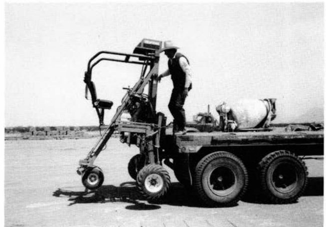
FIGURE 68—Use of the spyder forklift requires only one employee for delivering and unloading the adobe bricks at the building site. The Adobe Patch adobe yard, La Luz.
