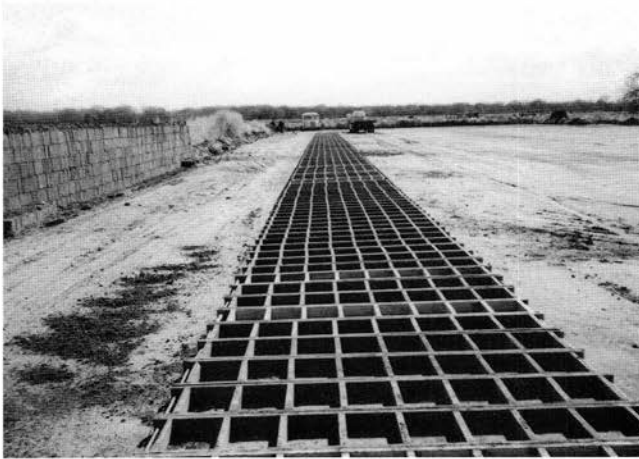
FIGURE 58—Ladder molding forms ready for filling. Rio Abajo Adobe Works adobe yard, Belen.
