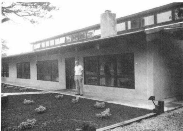
FIGURE 78—Hall Fouts of Gallup, with four untrained helpers and an Earth Press III machine, produced the walls of his solar pressed-earth-block house in five months beginning in November 1985.
