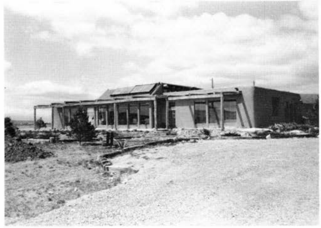
FIGURE 91—Huston house built with 16-inch-thick interior and 36-inch-thick exterior rammed-earth walls, Edgewood.
