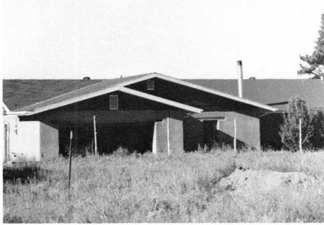
FIGURE 69—Narciso Garcia house built of 10,000 Porta Press pressed-earth blocks, Cedar Crest.
