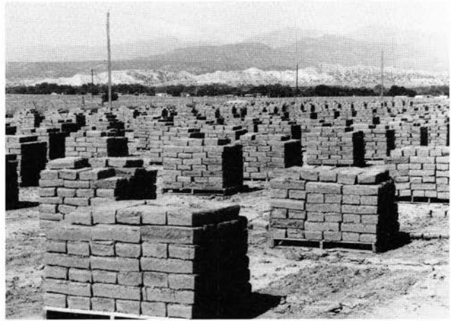
FIGURE 60—Dried and stacked adobe bricks. Adobe Factory adobe yard, Acalde.
