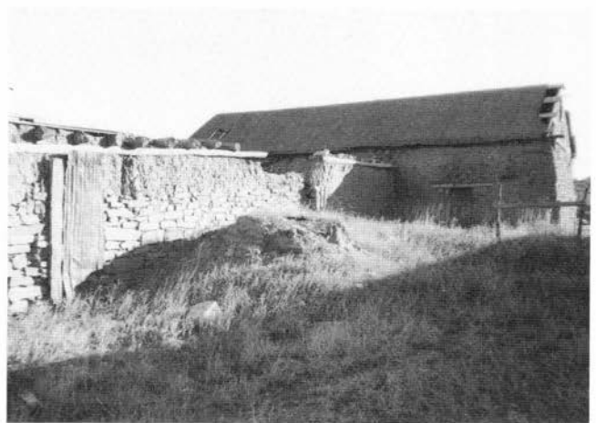
FIGURE 4—Old adobe and field-stone structure, San Jose.
