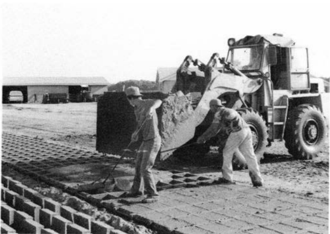
FIGURE 59—Pouring and raking the adobe-mud slurry into the ladder molding forms. Rio Abajo Adobe Works adobe yard, Belen.
