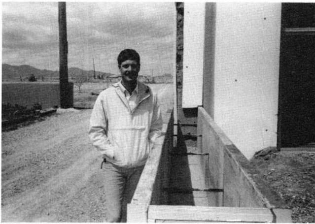
FIGURE 33—Stan Huston of Huston Construction Company standing by rammed-earth forms, Edgewood.
