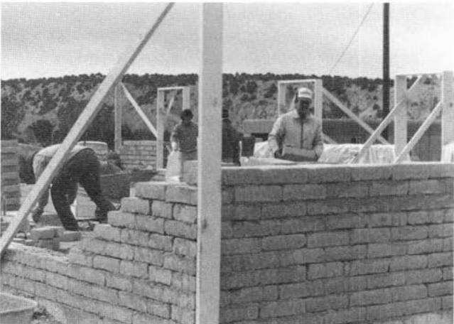
FIGURE 84—Pressed-earth-block house under construction. HUD building site, Nambé Pueblo.
