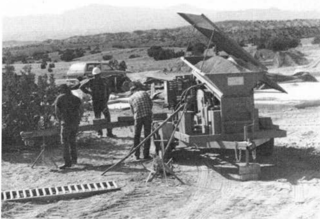
FIGURE 83—Pressed-earth-block production using the Goldbrick "5000" machine. HUD building site, Nambé Pueblo.
