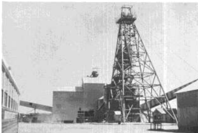
FIGURE 1—THE NO. 1 HEADFRAME AT THE IMC POTASH MINE NEAR CARLSBAD, NEW MEXICO.
