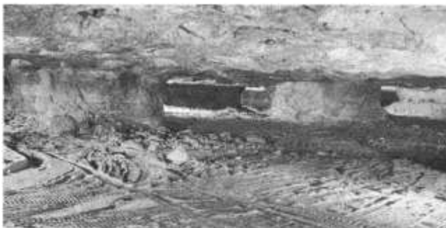
FIGURE 7—THIRTY-BY-50-FT PILLARS ARE LEFT FOR SUPPORT.
