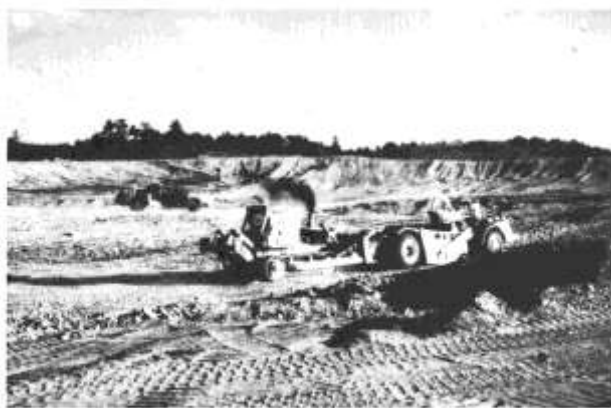
FIGURE 5—GREFCO WORKING PIT, NO AGUA.
