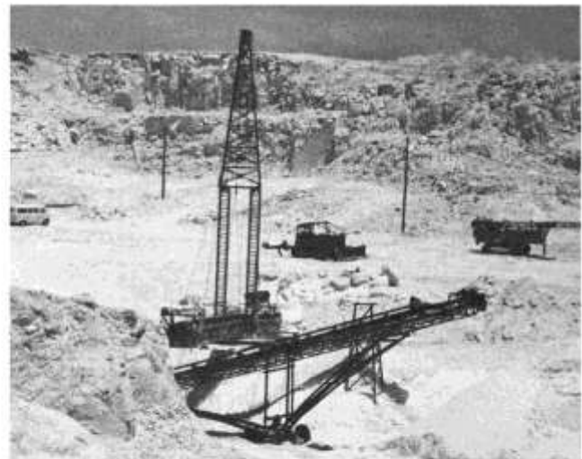
FIGURE 3—WHITE MESA MINE OF POMEROY, INC., LOCATED NORTHWEST OF ALBUQUERQUE. GYPSUM IS HAULED TO THE AMERICAN GYPSUM COMPANY WALLBOARD PLANT IN ALBUQUERQUE.
