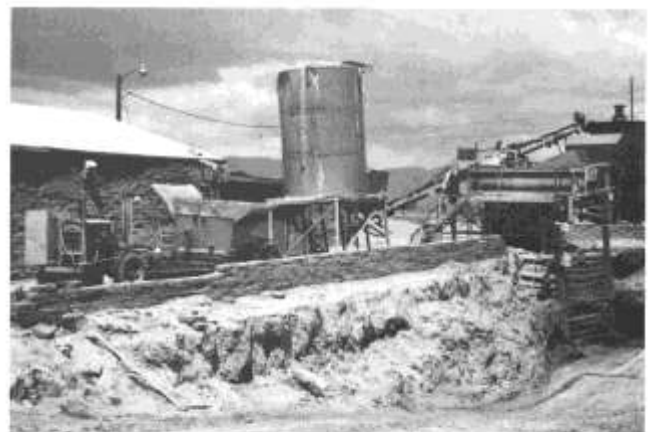
FIGURE 14—WATER AND OIL TANKS, PUGMILL, MUDPIT, AND CONVEYOR-BELT SYSTEM AT THE WESTERN ADOBE YARD IN ALBUQUERQUE.
