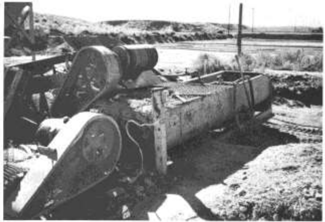
FIGURE 13—EXAMPLE OF A TYPICAL MIXING PUGMILL AT THE NEW MEXICO EARTH YARD IN ALAMEDA. After mixing soil, asphalt emulsion, and water, mud is dumped into the mudpit where it is removed by a Michigan Model 55 front-end loader for delivery to the wooden forms.
