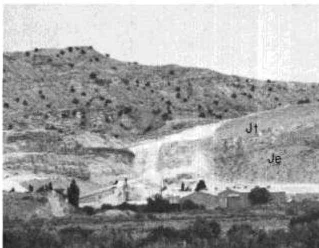
FIGURE 5—ROSARIO MINE AND WALLBOARD PLANT OF WESTERN GYPSUM COMPANY, LOCATED ALONG GALISTEO CREEK; Todilto Formation ( Jt ) overlying Entrada Sandstone ( Je ).
