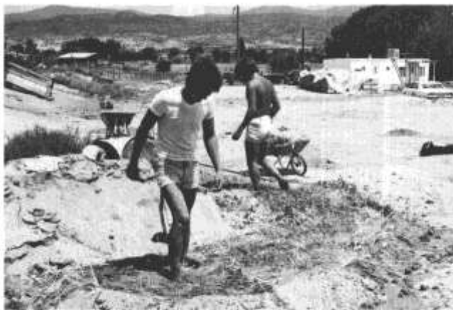
FIGURE 6—THE SYSTEM OF MIXING ADOBE MUD AND STRAW BY FOOT TREADING IN A MUDPIT IS THOUSANDS OF YEARS OLD. Photograph taken in Nambé, summer of 1980.
