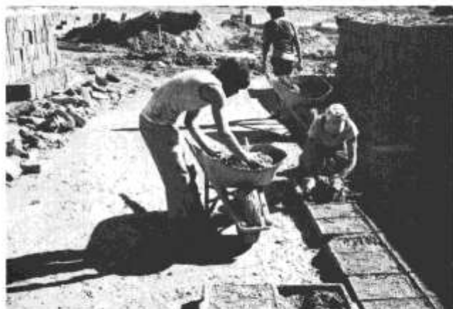
FIGURE 7—WHEELBARROWS DELIVER ADOBE MUD FROM THE MUDPIT WHERE IT IS PACKED INTO WOODEN FORMS THAT MOLD FOUR BRICKS AT A TIME. Photograph taken in Santa Fe, summer of 1980.
