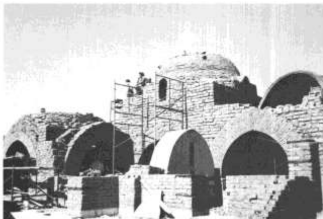
FIGURE 4—THE DAR AL-ISLAM MOSQUE PROJECT IN ALBUQUERQUE WAS UNDER CONSTRUCTION IN 1980 USING SEMISTABILIZED ADOBE BRICKS. Note arch and dome structures that are common in North Africa.
