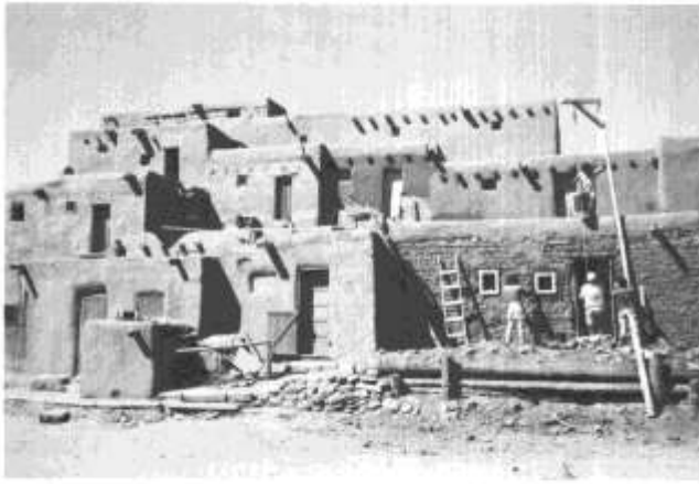
FIGURE 3—TAOS PUEBLO IS AN EXAMPLE OF PUEBLO ARCHITECTURE OF FIVE STORIES THAT HAS BEEN CONTINUOUSLY OCCUPIED FOR OVER 900 YRS. Photograph taken in August, 1980 during the annual replastering of the Pueblo.
