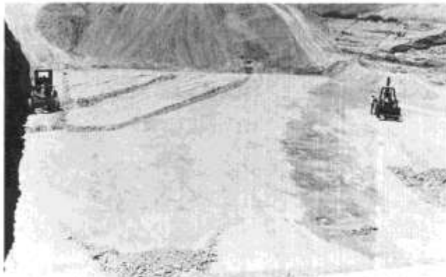
FIGURE 13—A PALEOCHANNEL (DARK-COLORED AREA NEXT TO BACKHOE) THAT CUTS THROUGH UNMINED, HIGH-GRADE BED AT THE BOWIE CHABAZITE DEPOSIT. Direction of flow is from the bottom of the photograph toward the top.
