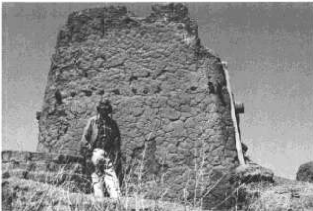
FIGURE 2—JESUS MERMEJO OF PICURIS PUEBLO STANDING NEXT TO THE OLD PUEBLO STRUCTURE BUILT OF PUDDLED ADOBE BETWEEN 1250 AND 1300 A.D. Site visited by the Spanish conquistador Juan de Oñate on July 13, 1598.
