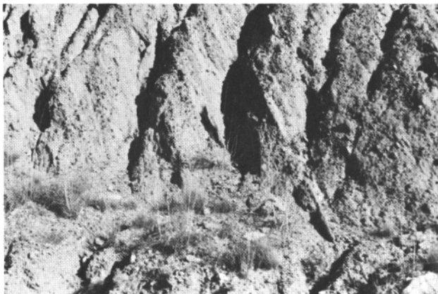
FIGURE 18—STEEPLY DIPPING SANTA FE GRAVEL IN NORTH SIDE OF RAILROAD CUT SEC. 10, T. 7 N., R. 2 W. Exposure is about 50 ft east of the Santa Fe fault where Jurassic beds are upthrown on the west.
