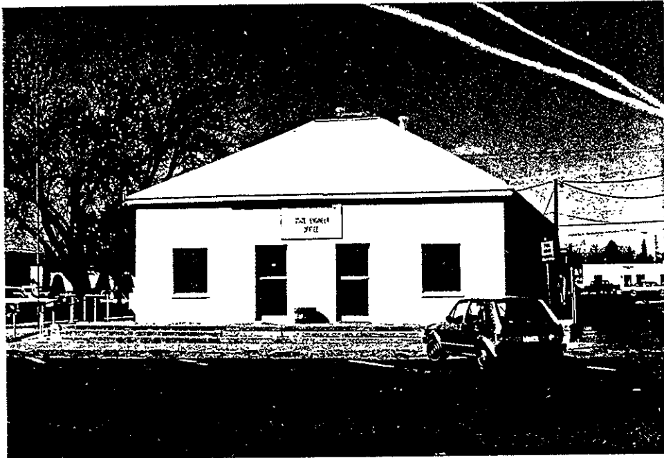
Figure 3. State Engineer Office, Deming
