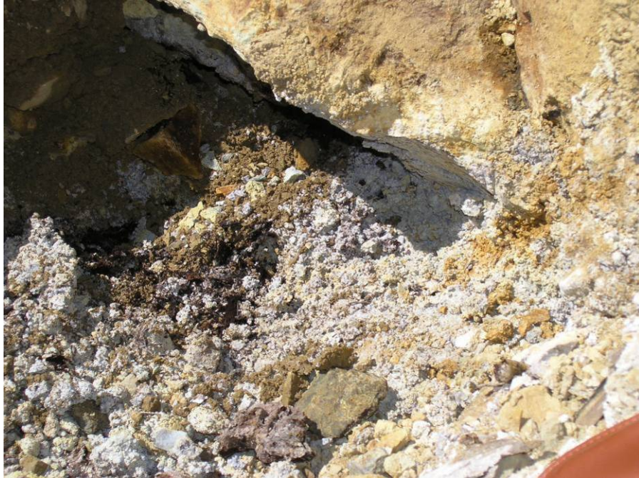
FIGURE 23. Surficial zones of white to yellow-brown soluble salts, gypsum, and jarosite on GHN.
