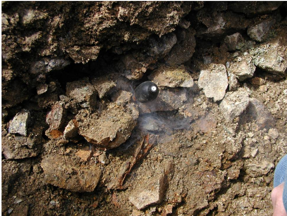
FIGURE 129. Photo of venting gases in GHN using a smoke bomb (GHN-LFG-0003-H019).
