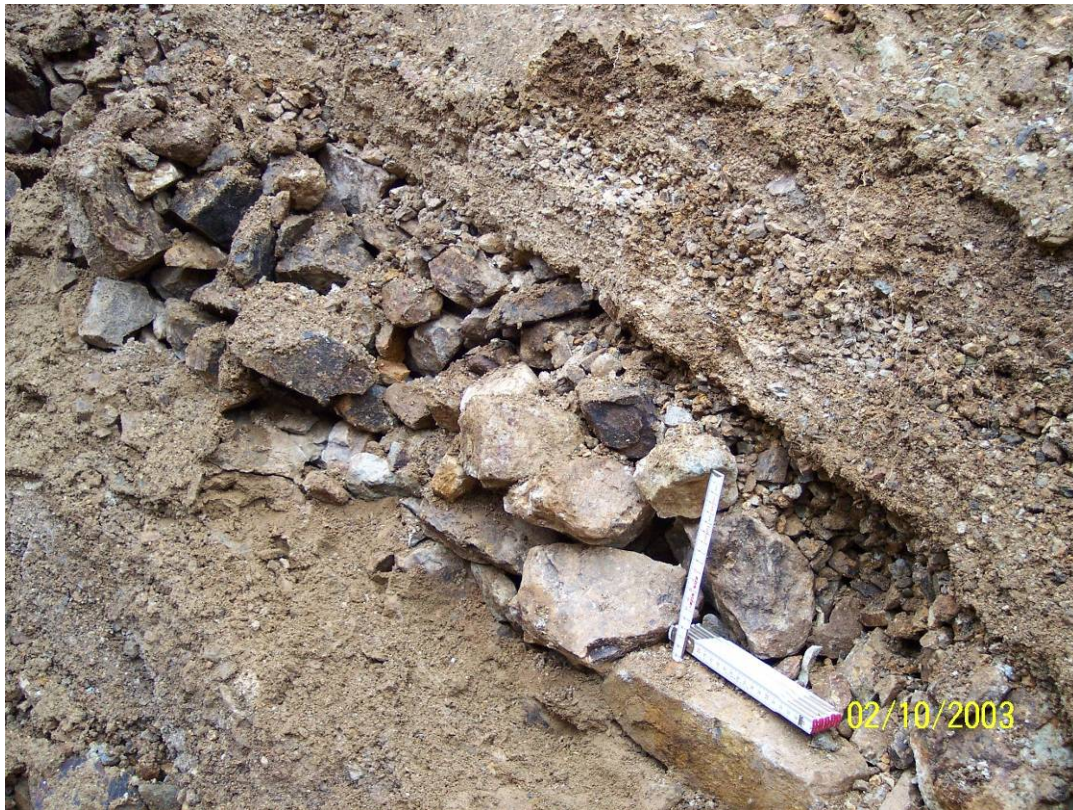
FIGURE 31. Toe of GHN rock pile (2/10/03).
