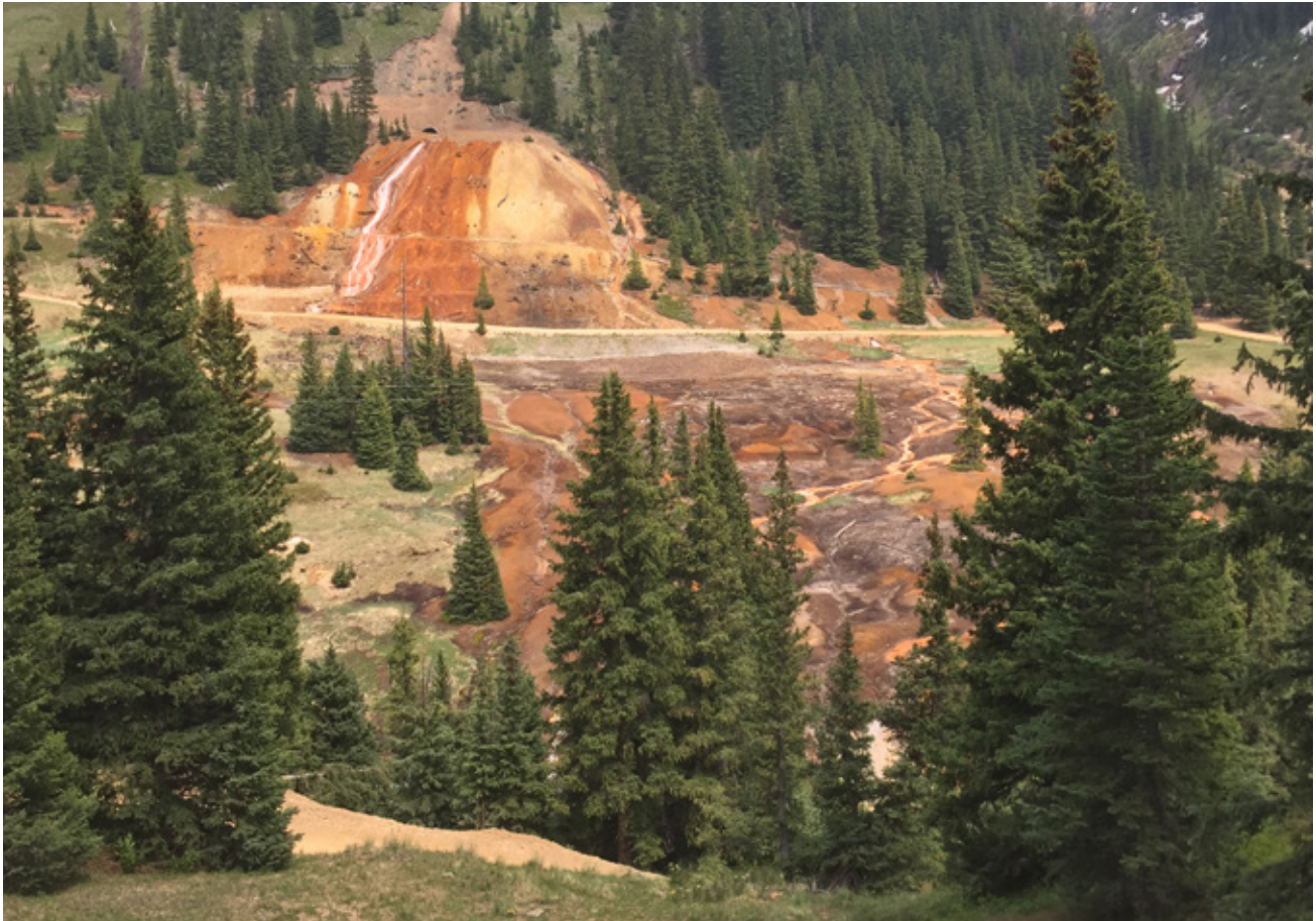
Water is flowing out of the Red and Bonita Mine over orange stained waste rock piles. These waters contribute to Cement Creek, which flows into the Animas River near Silverton, Colorado.
