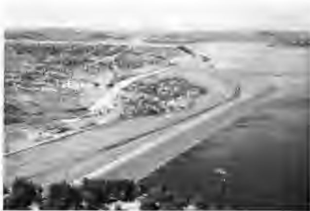
Figure 9—NAVAJO DAM AND RESERVOIR, 18 mi north of Aztec; view to north.
