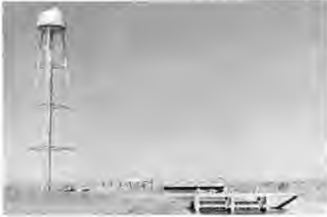
Figure 100—TYPICAL CONVEYANCE CANAL, PUMPING STATION, AND WATER TOWER USED TO DISTRIBUTE WATER IN NAVAJO INDIAN IRRIGATION PROJECT. Photo taken in block 1, west of NM-44 and south of Bloomfield.
