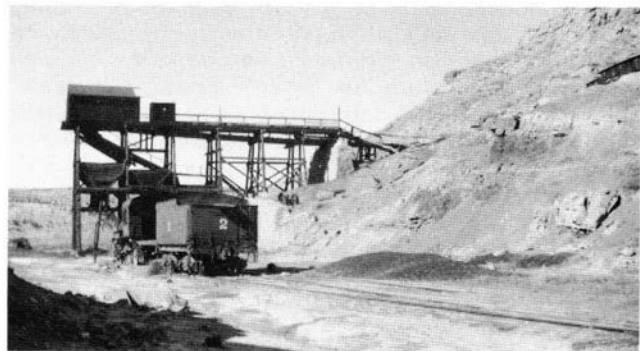
FIGURE 176—The tippie and loading dock at the San Juan mine. Note the stranded engine and tender, which probably belonged to Santa Fe Northwestern Railroad. A cloudburst had washed out several trestles, and they were never repaired. Photo by J. J. Bourquin, February 10, 1937.
