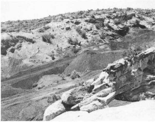
FIGURE 100—Bulldozing done in about 1979 at the Enterprise-Jones-Neff mine, which exposed the 30-ft bed of coal amidst the old mine openings (view is S15°E). The loose coal on the exposed outcrop provides an ideal condition for spontaneous combustion in the spoil pile; a crop fire could be created that would be difficult or impossible to extinguish. Photo by H. B. Nickelson, 1979.
