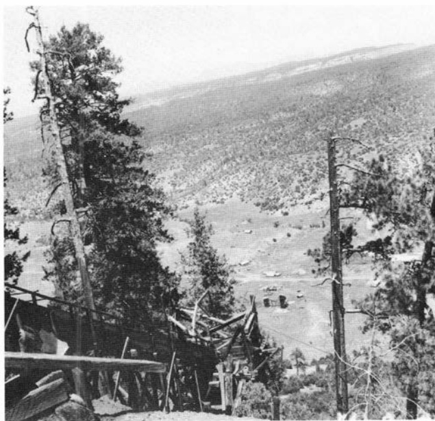
FIGURE 117—View looking north from the Caranta No. 4 mine chute. The chute connected to the No. 1 mine bin where the coal was transported by aerial tramway to the smaller of the two bins on the valley floor. Photo by H. B. Nickelson, 1979.
