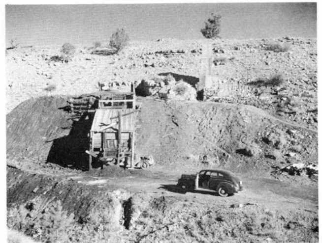
FIGURE 119—The portal and chute of the original Erler (Rainbow) mine. The chimney to aid ventilation is directly under the tree on the horizon. The black car in the foreground was the government car used by Mr. Allport. Photo by R. H. Allport, September 27, 1943.
