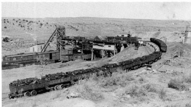
FIGURE 5—The loading facilities at Southwestern mine. The loaded cars in the foreground were each uncoupled, weighed on a scale, and dumped in a small bin over the shaker screens. The dumping procedure consisted of placing the car on the dumping mechanism, opening the front of the car, and releasing the dump so the car would tip, unloading the coal onto the screens. The shaker screens sized the coal in lump, engine coal, and slack, and it was then loaded directly into railroad cars. The boxcars on the left track received the lump coal; engine coal was loaded on the middle track, and slack coal was loaded over the near track, both in open cars. Photo by H. C. Stacher, April 5, 1933.
