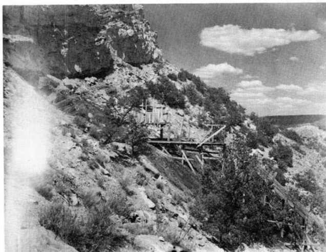
FIGURE 194—Hoist house, tippie, and chute built by Mr. Jack in the steep hillside of the Jack prospect. Photo by R. H. Allport, June 14, 1946.
