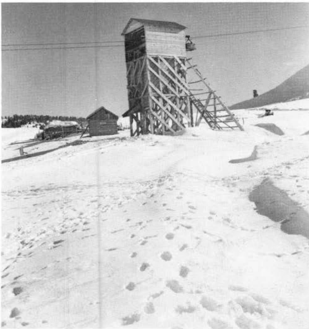
FIGURE 114—This partly constructed storage bin on the valley floor was for the coal mined from the Caranta No. 2 and No. 3 mines. The bucket and cable to the right of the bin are part of the tramway for the storage bin for the No. 1 and No. 4 mines. Photo by R. H. Allport, winter 1943–44.
