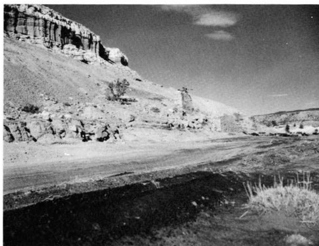
FIGURE 178—The foundation of the tippie at the San Juan mine and the terrace formed by the USBM to control the mine fire. Photo taken in February 1951.
