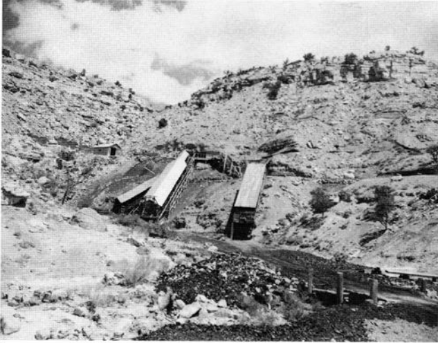
FIGURE 198—Surface facilities at the Tohatchi mine. Photo by R. H. Allport, April 25, 1947.
