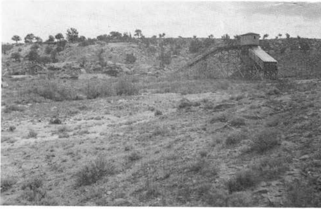
FIGURE 16—The tippie and coal chute, constructed by Peter Pavioni, at the Black Star mine. Photo by J. J. Bourquin about 1931.
