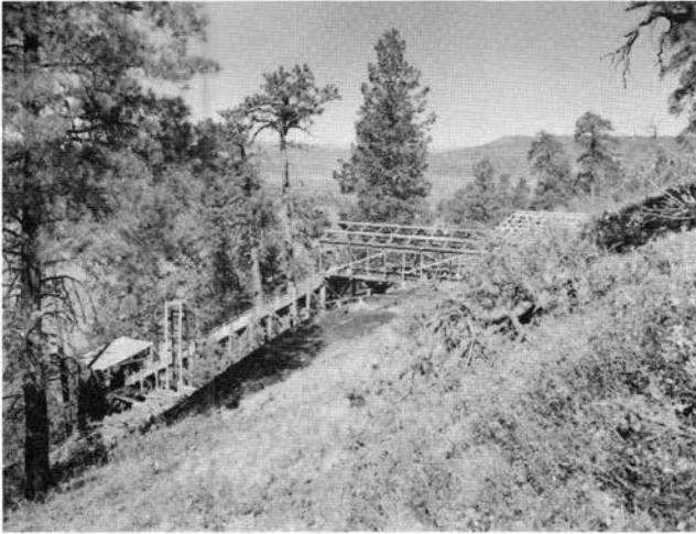
FIGURE 113—The Caranta No. 1 and No. 4 mines surface facilities, which were constructed in 1943. The coal from the No. 2 mine was dumped over a tippel into the chute to the No. 3 mine bin where it was combined with the No. 3 mine coal. The coal was then transported from this bin by a 2,900-ft-long aerial tramway to a larger bin (Fig. 114) on the valley floor. Photo by R. H. Allport, 1945.
