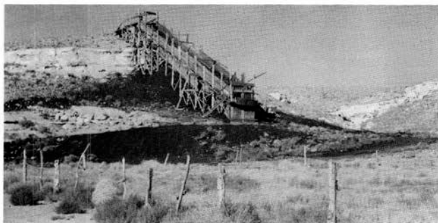
FIGURE 94—Mine tibble and storage bins at the Silva mine. Photo by R. H. Allport, October 24, 1942.
