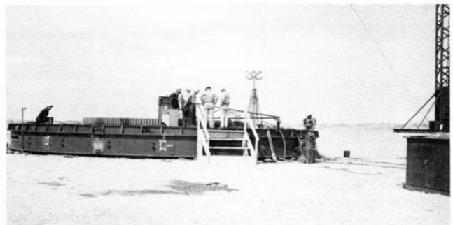
FIGURE 75—The Marion model 5323 shovel being reassembled at Utah's Navajo mine assembly yard. This shovel, carrying a 22-yd 3 dipper, was moved from the company's worked-out Ozark Philpott operation in Arkansas. It was used to start the first box cut in the Dodge pit while the Marion 7900 dragline was being constructed, and then it aided the dragline in the early stripping operations. Later it was used to load coal from the pits, but it was not too successful because of its awkward size. It was eventually retired and sold. Photo by H. B. Nickelson, summer 1961.
