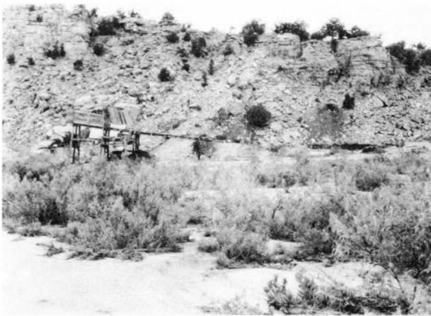
FIGURE 170—Simple tippie and chute constructed to handle coal from the development workings of the Weil slope at the Sandoval Coal Company mine. Photo by J. J. Bourquin, April 26, 1929.
