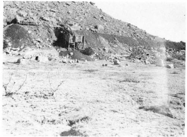
FIGURE 164—White Ash mine; photo was taken soon after Mr. Wetherill had made application for a lease. Photo by J. J. Bourquin, April 1929.
