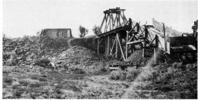
FIGURE 14—The shaft and the coal chute at the Cardo mine about 1924. The building served as a hoist house, shop, and tool storage shed. The coal on the ground is slack. Photo by engineers from U.S. Geological Survey.
