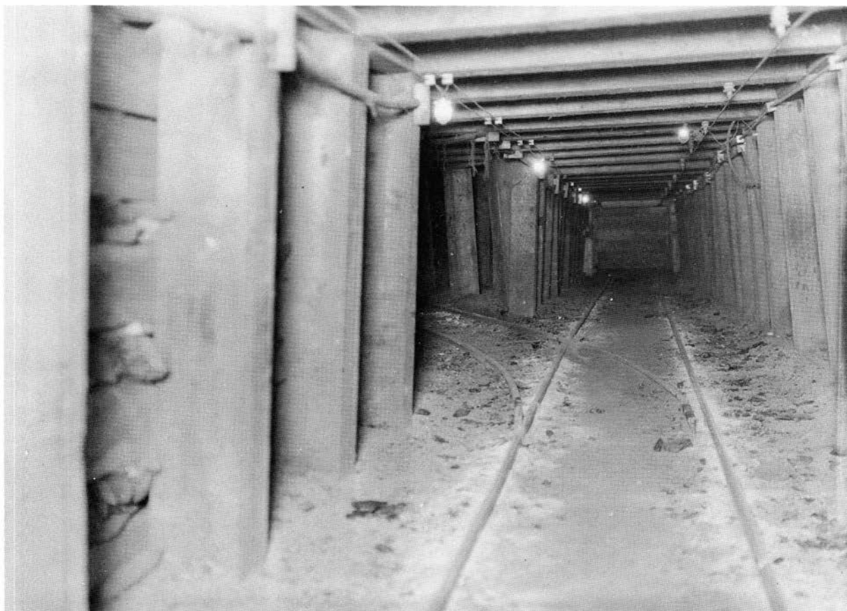
FIGURE 45—Underground entry showing the main line timbering in the Navajo No. 5 mine, Gallup, New Mexico. Photo courtesy of John Kleiner; NMBMMR photo #686.
