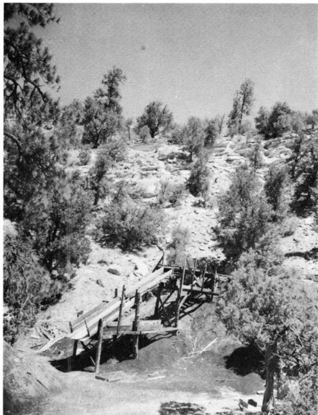
FIGURE 146—The crude tippie and chute at the Kern mine. Photo by R. H. Allport, June 14, 1946.
