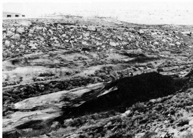
FIGURE 25—View looking N70°W of the old mine dumps from the Black Diamond et al. mines at Diamond gulch. The mine portals were all above this rim to the north. A trestle was built from the rim across the gulch; the coal bins and railroad loading dock were under the trestle, and the refuse was dumped from the trestle to form these dumps. Note the water tower on the horizon and the new school on the left. Photo by H. B. Nickelson, 1979.
