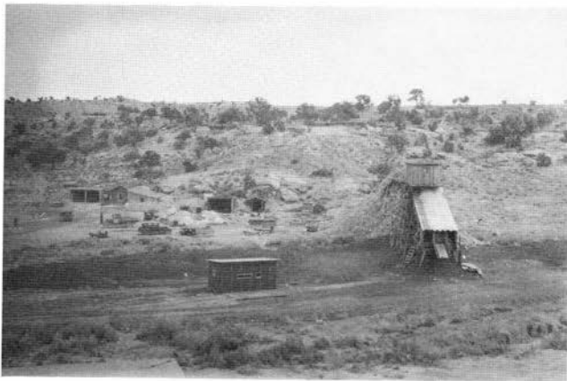
FIGURE 17—Black Star mine surface facilities, which were constructed by Peter Pavioni. Photo by J. J. Bourquin, March 26, 1933.
