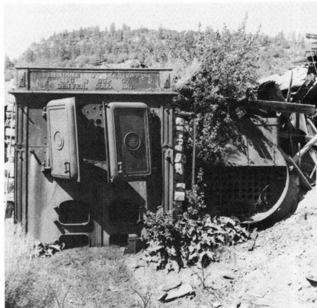
FIGURE 109—The remains of the old steam boilers used to provide electric power for the mine pump, hoist, and other electric power needs at the Luchetti mine. Photo by H. B. Nickelson, 1979.
