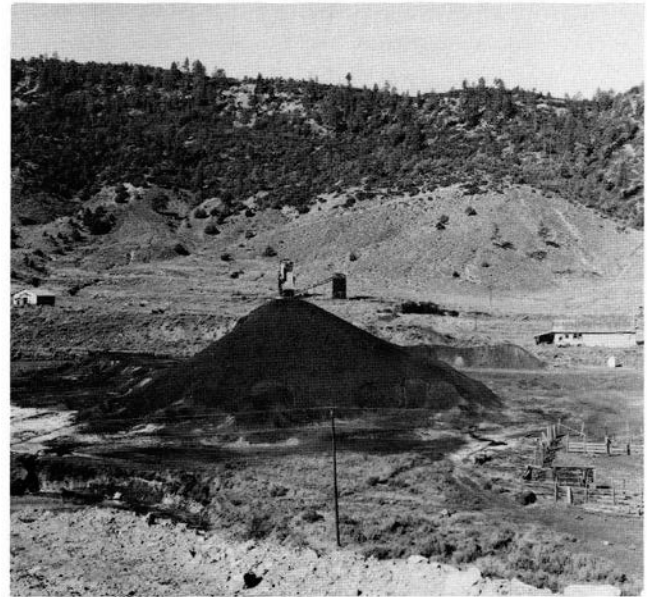
FIGURE 110—The old Monero mine site showing the screening or refuse dump, the old Caranta store and Post Office, and the railroad loading dock. The structure over the top of the spoils pile was the base of the aerial tram and storage bin built by the Carantas for their mines at the top of the ridge. Photo by H. B. Nickelson, 1979.
