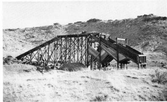
FIGURE 90—The George Simpson No. 12A mine surface facilities. These were the best tippel and bins used at the Hogback mines; this tippel later burned. Photo by R. H. Allport, October 7, 1949.
