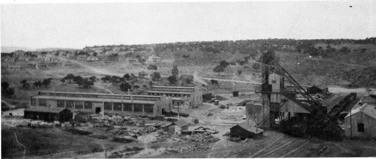
FIGURE 42—Surface facilities at Navajo No. 5 mine, October 15, 1922. To the left are the electrical shop, warehouse, and machine shop. To the right are the headframe and hoist house. The town is in the background. Photo courtesy of John Kleiner; NMBMMR photo #700.
