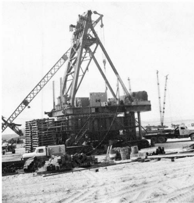
FIGURE 75—The Marion model 5323 shovel being reassembled at Utah's Navajo mine assembly yard. This shovel, carrying a 22-yd 3 dipper, was moved from the company's worked-out Ozark Philpott operation in Arkansas. It was used to start the first box cut in the Dodge pit while the Marion 7900 dragline was being constructed, and then it aided the dragline in the early stripping operations. Later it was used to load coal from the pits, but it was not too successful because of its awkward size. It was eventually retired and sold. Photo by H. B. Nickelson, summer 1961.
