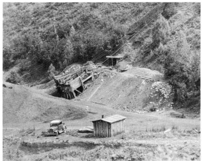
FIGURE 133—The surface facilities of the Belino-Peisker mine, showing the large pile of slack coal stored beyond the storage bin and cables that anchored the chute and bin to the hillside. Photo by J. J. Bourquin, September 2, 1937.
