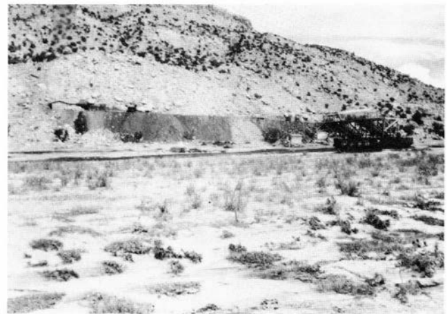
FIGURE 166—White Ash mine railroad loading facilities and the portal. Photo by C. C. Mather, September 8, 1930.
