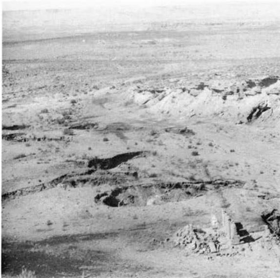
FIGURES 98a and b—Telephoto pictures of the surface subsidence at the Caudell mine. Photos by R. H. Allport, September 30, 1943.
