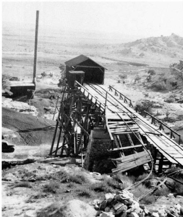
FIGURE 177—The tippie and loading dock of the San Juan mine. Photo taken on October 28, 1942.
