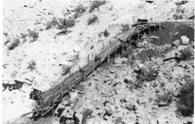
FIGURE 200—The chute constructed about 1960 at the new portal of the Martin mine. Photo by H. B. Nickelson, April 2, 1962.
