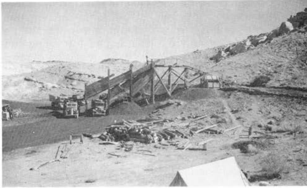
FIGURE 89—A common type of tippel at the Hogback mines; this one was at the Hogback No. 12 mine. Photo by R. H. Allport, October 6, 1944.
