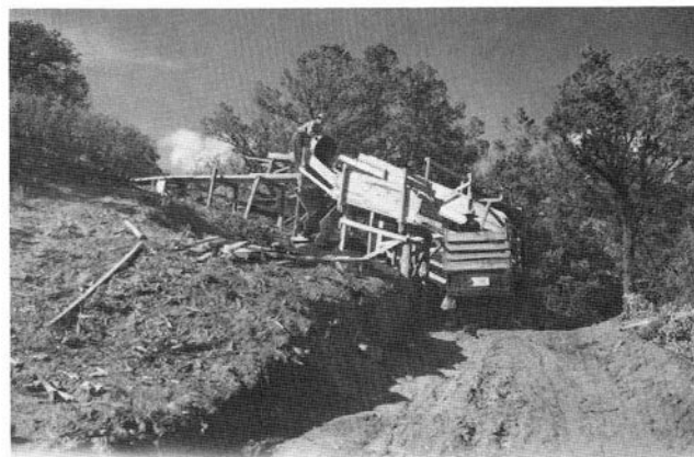
FIGURE 195—Small tippie, wheelbarrow, and wash tub used to operate the Amick prospect. Photo by R. H. Allport, October 23, 1944.
