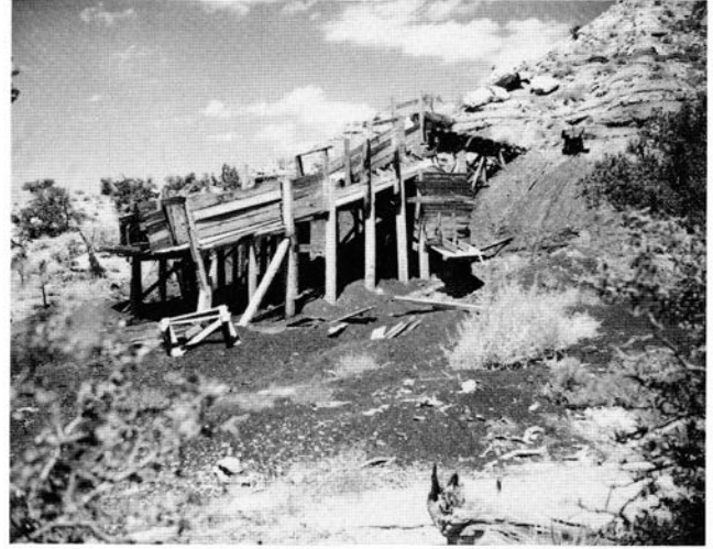
FIGURE 216—Abandoned tippie and coal chute at the Smouse prospect. Photo by R. S. Fulton, August 15, 1949.
