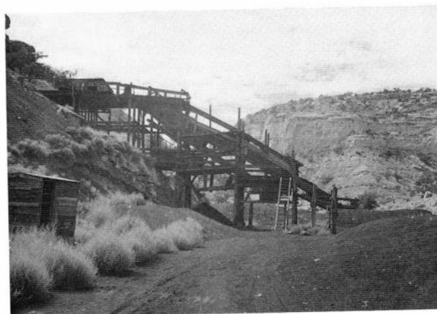
FIGURE 185—Tippie used for the Sackett operations at the Anderson-Sackett mine. Photo by R. D. Reeder, January 8, 1942.
