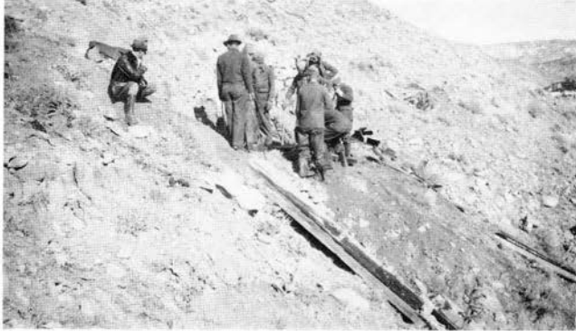
FIGURE 174—Superintendent Evan Carron and laborers from the Soil Conservation Camp No. 7 sealing the air shaft in order to control the fire at the San Juan mine. Photo by J. J. Bourquin, February 9, 1937.
