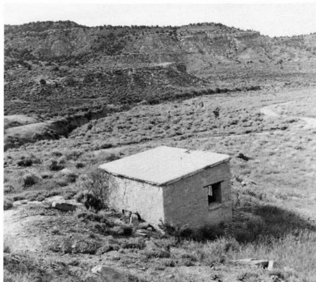
FIGURE 38—Powder house at the Gallup-Gibson mines. These well-constructed stone buildings, found near the larger coal mines, have survived. They were used to safely store and dispense explosives as they were needed underground.
