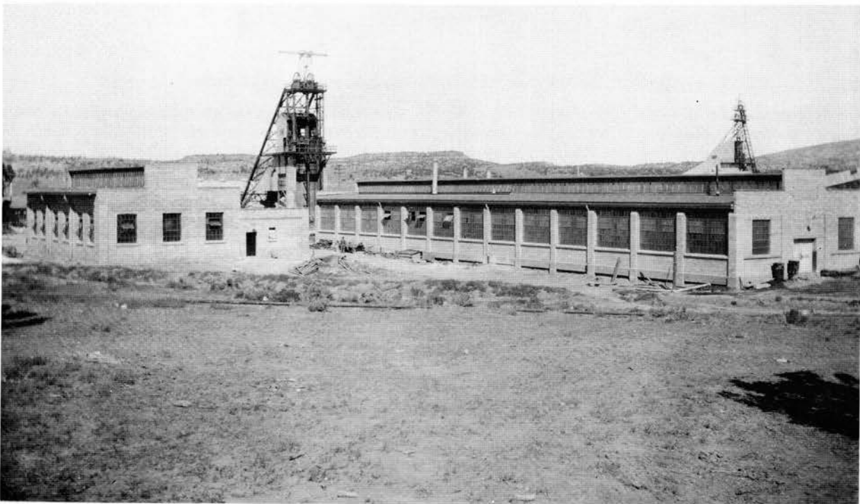
FIGURE 44—Shaft, tippel, and buildings at Navajo No. 5 mine, October 15, 1922. Photo courtesy of John Kleiner; NMBMMR photo #693.
