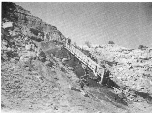
FIGURE 66—Coal chute at the Padilla-Maestas prospect. Photo by R. H. Allport, October 24, 1944.
