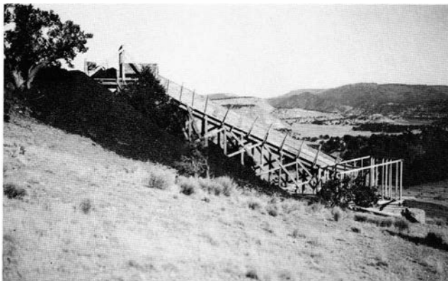
FIGURE 152—Tippie and chute at the Sunny Slope mine, which were built before the issuance of the lease. Photo by R. D. Reeder, December 13, 1938.
