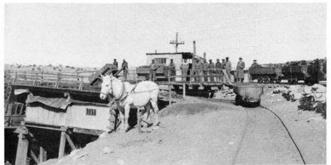
FIGURE 7—The white mule is waiting to pull empty cars back to the mine entrance of the Southwestern mine where they will be coupled to the main haulage rope to be lowered back into the underground for reloading by the miners. Photo by H. C. Stacher, April 5, 1933.
