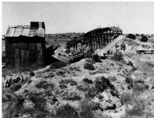
FIGURE 57—A view of the Marquez mine showing the fan house in the left foreground; the fan sits over a vertical shaft. The tippie and loading bin are in the center background. The incline is just beyond the truck. The waste was dumped under the tippie. Photo by H. B. Nickelson, 1979.
