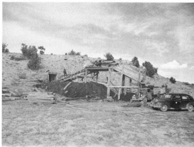
FIGURE 189—Portal, hoist, and small chute at the Yarbrough mine. Photo by R. H. Allport, October 22, 1944.
