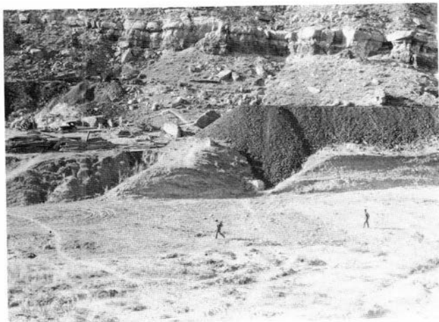
FIGURE 183—Coal stockpile at the Anderson mine before the railroad spur connection with the main line was completed. This coal fired and was destroyed. Photo by C. C. Mather, December 13, 1929.
