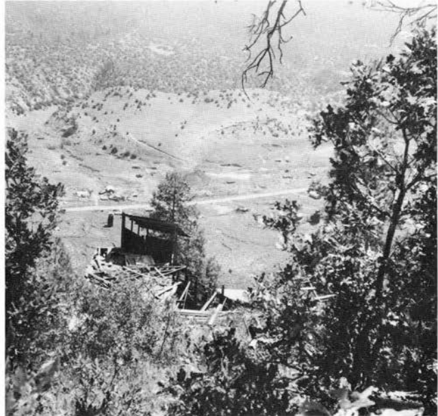
FIGURE 115—The old tippel, chute, and bin at the Caranta No. 5 mine. This bin was the loading dock for the aerial tramway, which was unloaded in a bin at the bottom of the hill. The latter bin is visible to the left of the left edge of the shed. Photo by H. B. Nickelson, 1979.
