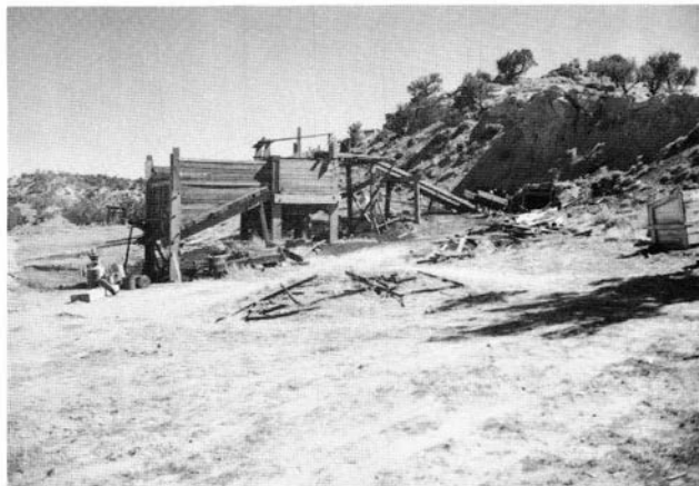
FIGURE 188—Tippie, coal bin, and portal at the Tonopah mine. Photo by R. H. Allport, March 19, 1948.
