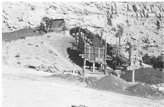
FIGURE 181—Tippie at the Luciani Peacock No. 3 mine. This tippie was also used to accommodate the coal from the Peacock No. 4 mine on state land via track laid between the two portals. Photo by R. D. Reeder about 1940.
