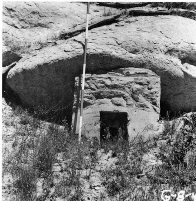
FIGURE 37—Stone and concrete structure at the Weaver mine. The structure, which enclosed a vent pipe, was used to take air samples to check the underground atmosphere in order to monitor the fire in the old mine workings. Photo by H. B. Nickelson, 1979.
