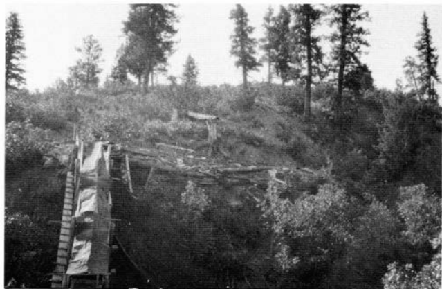
FIGURE 140—Lobato prospect; part of the chute is covered with sheet metal to keep the coal dry. Photo by C. L. Duer, September 1928.
