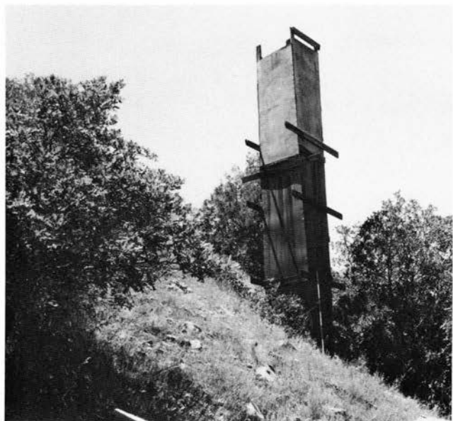
FIGURE 116—Ventilation chimney at the Caranta No. 4 mine. In this method of mine ventilation a fire built at the base of the chimney created heat that rose and pulled the air in the mine out through the chimney. Photo by H. B. Nickelson, 1979.
