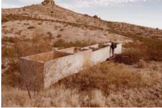
FIGURE 40. Leach tanks at the Canon mine, Tres Hermanas district (V. T. McLemore, photo).
