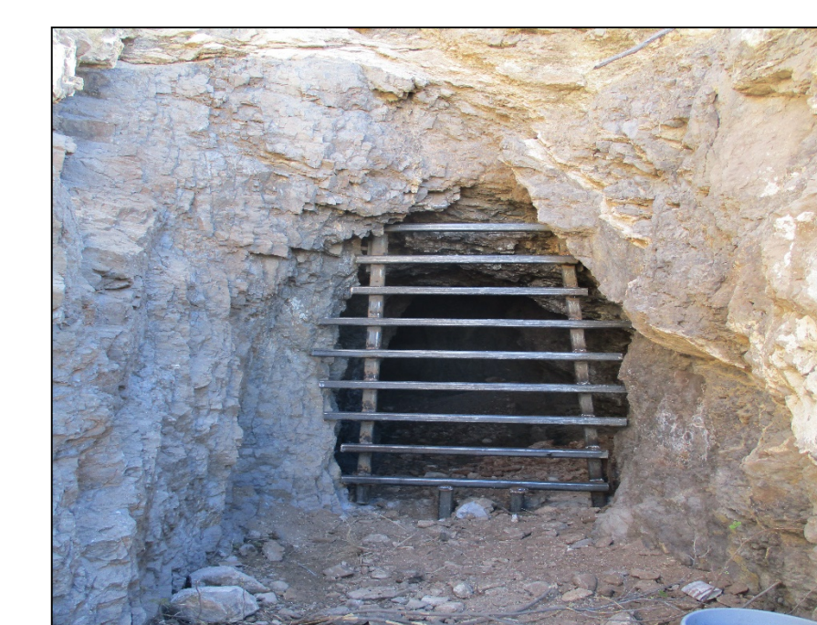
Bat gate in adit.
