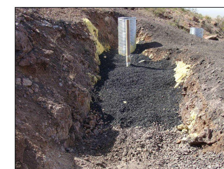
Backfilling the mine shaft.
