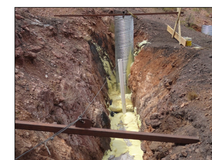
Applying polyurethane foam.
