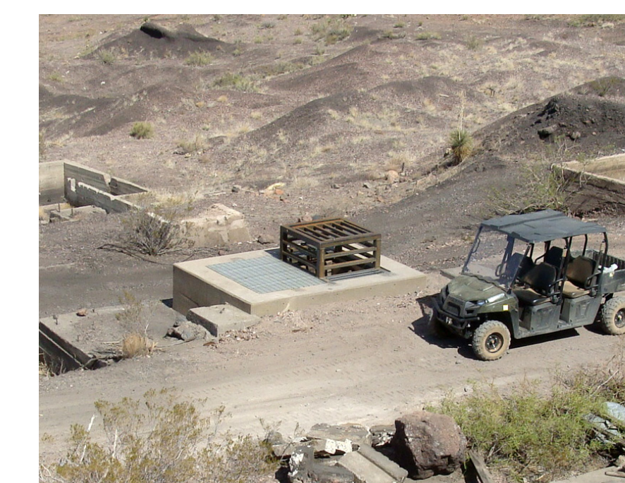
Cupola installation that preserves historical integrity.
