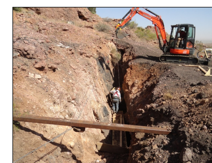
Constructing support for the riser.
