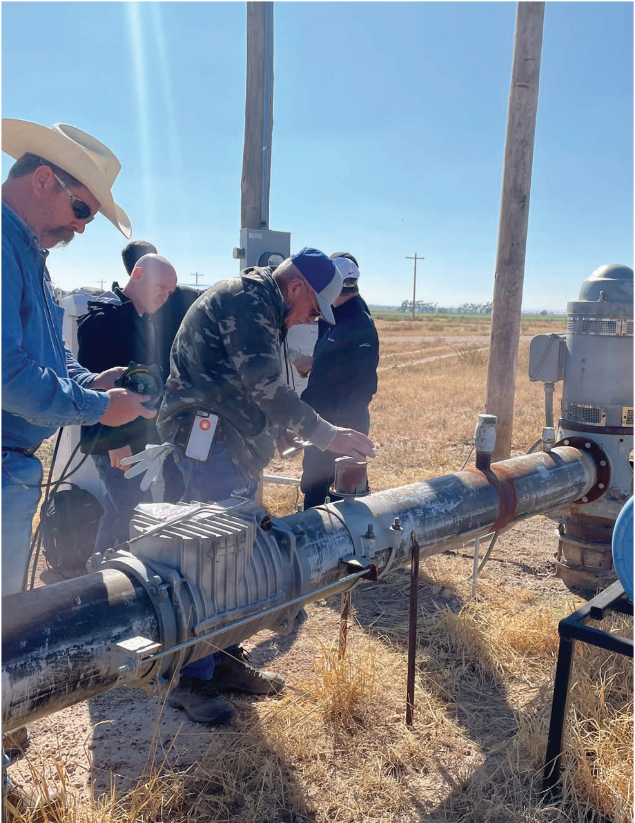
An irrigation well in the Pecos Valley being equipped with a new meter with telemetry to help track pumping volume, which, when used with groundwater levels, provides a more complete picture of aquifer behavior and trends.
