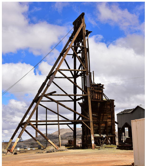
A modern (March, 2019) view of Florence Mine and its remaining headframe.
