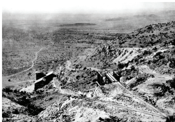
View of Western Mineral Product Co.'s mill looking north, circa 1916. Photograph courtesy of Wally Clark, St. Joe American Corp., Tucson AZ, New Mexico Bureau of Geology and Mineral Resources, Historic Photograph Archives, Socorro, NM 87801.
