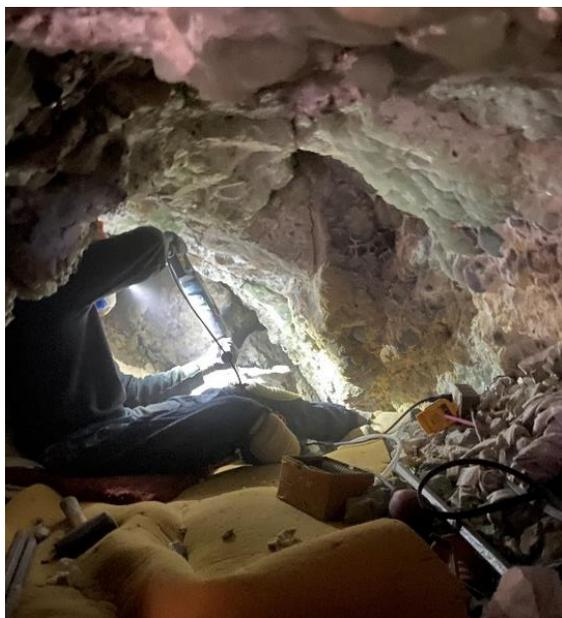
*Figure 2: Bradley Culebro drilling feather and wedge holes with an electric hammer drill to split a large slab in the Ice Cream Scoop pocket. May 13, 2023. Mike Sanders photo.*
