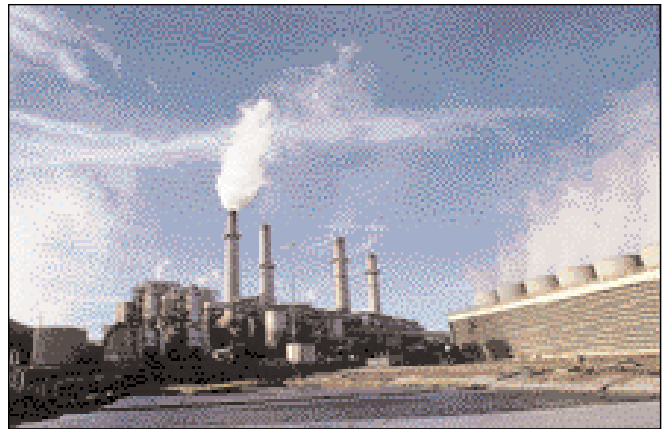
Public Service Company of New Mexico's San Juan Generating Station, north of Waterflow.
