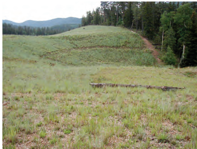
The Las Conchas mine following reclamation. The site was contoured and seeded with native vegetation so that it blended in with the surrounding ecosystem after only a few years of average rainfall.
