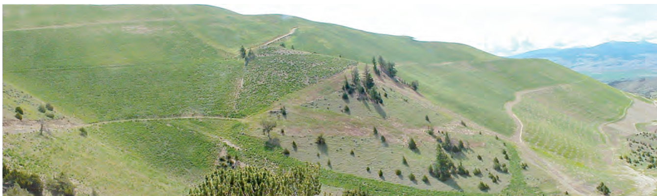
Modern mine reclamation often includes extensive areas of uniform slopes, with slope breaks/benches and constructed drainageways.
