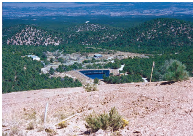
This catchment pond at the Ortiz mine in northern New Mexico was built to prevent mine drainage from entering surface streams.
