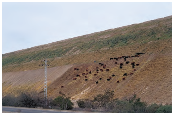
Reclamation and slope stabilization on tailings at the Miami mine in Arizona. The cows are grazing on the newly reclaimed slope to the right.
