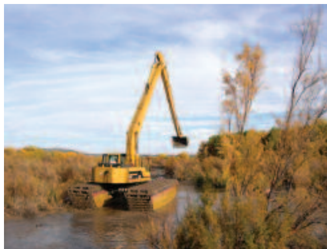
An amphibious excavator clearing the Tiffany plug in fall 2005.
