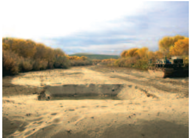
A close up of the sediment plug near Tiffany in fall 2005. The excavation in the center of the photo has revealed the location of the water table, several feet below the surface of the plug.
