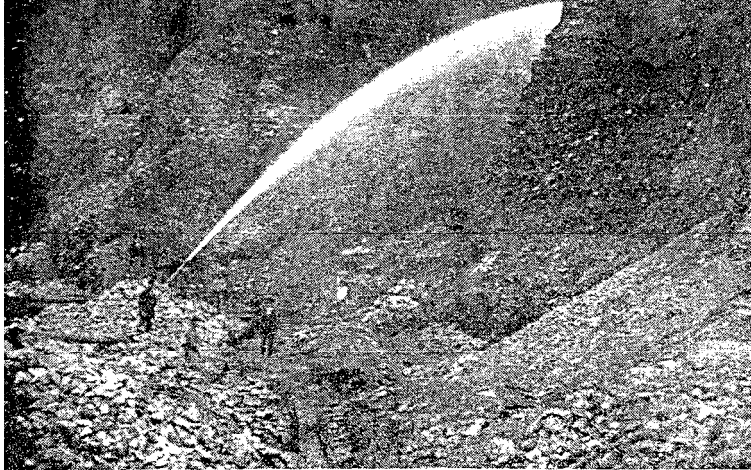
Hydraulicking at Elizabethtown, about 1900.
