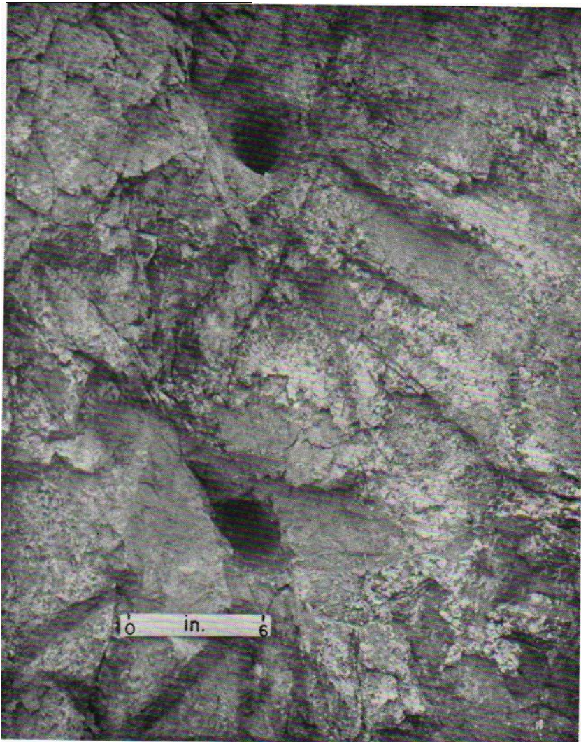
Figure 8 CRATERLESS HOLES SHOT INTO ALTERED QUARTZ MONZONITE WITH 4- INCH DIAMETER CAST IRON LINERS
