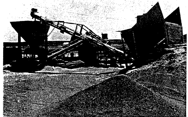
B—SCREENING EQUIPMENT, STORAGE BINS, AND CONVEYOR SYSTEM.
