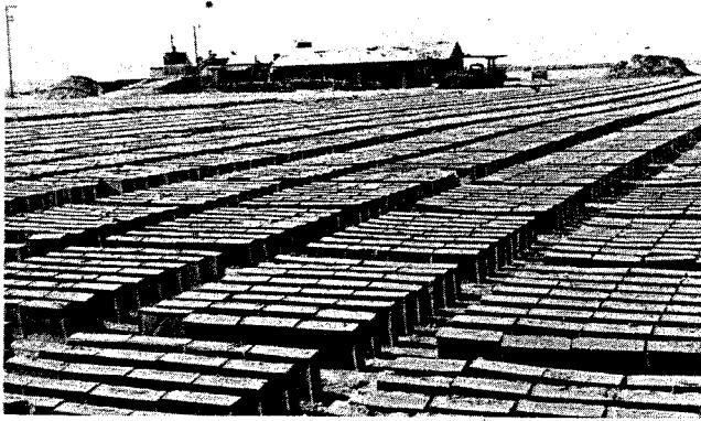
FIGURE 81—WESTERN ADOBE YARD, ALBUQUERQUE.
