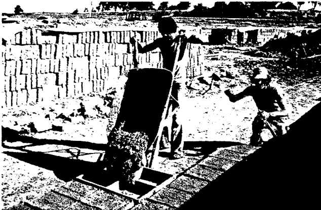
A-ADOBE MUD IS DUMPED INTO WOODEN FORMS.
