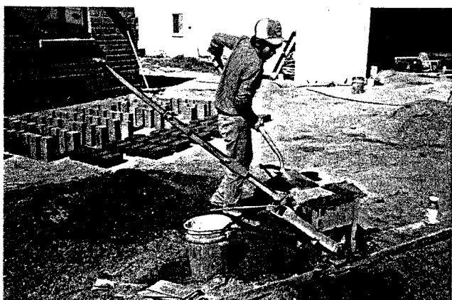
B-ADOBE SOIL IS SHOVELED INTO CINVA-RAM MOLD AND TAMPED WITH SHOVEL.
