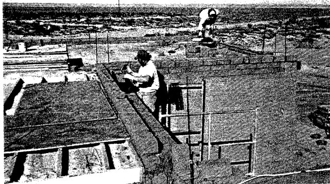
FIGURE 78-LAYING A DOUBLE WALL OF CINVA-RAM-MADE PRESSED ADOBES AT THE W. S. CARSON HOUSE IN COLUMBUS.
