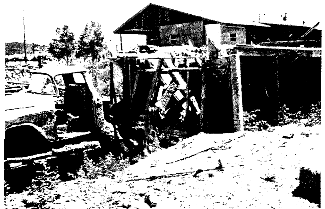
A-MATERIAL HOPPER AND POWER EQUIPMENT.
