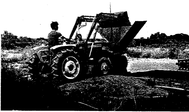
A-FRONT-END LOADER LOADING CEMENT-MIXER HOPPER WITH ADOBE SOIL.
