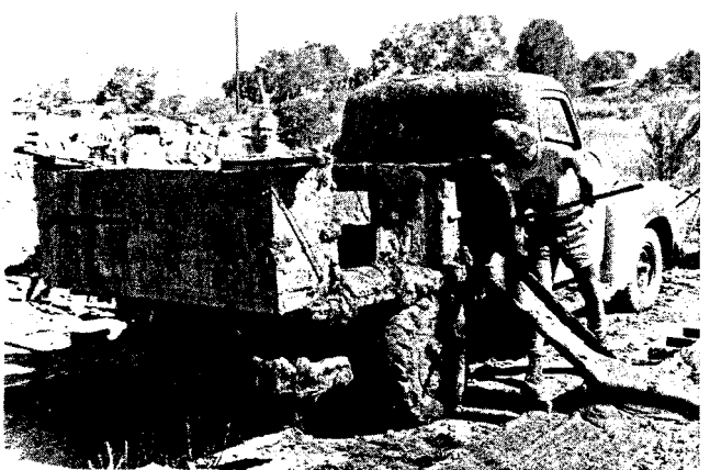
B-SIDE SLOTS ON MUD VEHICLE ARE OPENED, AND MUD FLOWS INTO WOODEN MOLDING FORMS ON EACH SIDE OF TRUCK.
