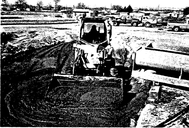
E-FRONT-END LOADER REMOVING MUD FOR DELIVERY TO WOODEN MOLDING FORMS IN DRYING YARD.
