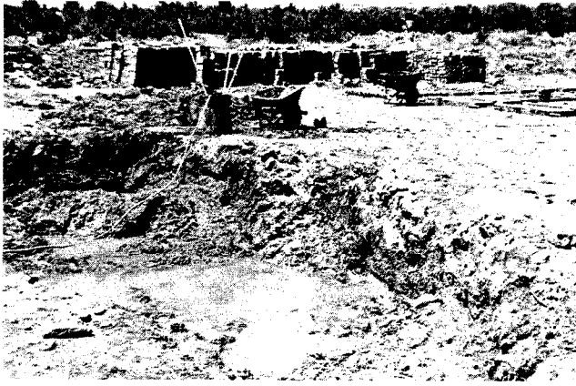
A-MUDPIT EXCAVATED BY BACKHOE AND USED TO MIX WATER, STRAW, AND ADOBE SOIL.
