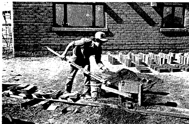
A-ADOBERO PLACES FLAT STEEL PLATE IN BOTTOM OF CINVA-RAM MOLD.
