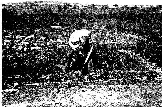
B-AFTER SIDE AND END CUTS HAVE BEEN MADE DOWN TO ROOT LEVEL. TERRÓN IS WEDGED FROM SOD.
