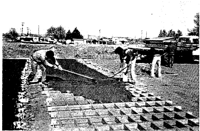
G-ADOBEROS RAKING ADOBE MUD INTO MOLDING FORMS.
