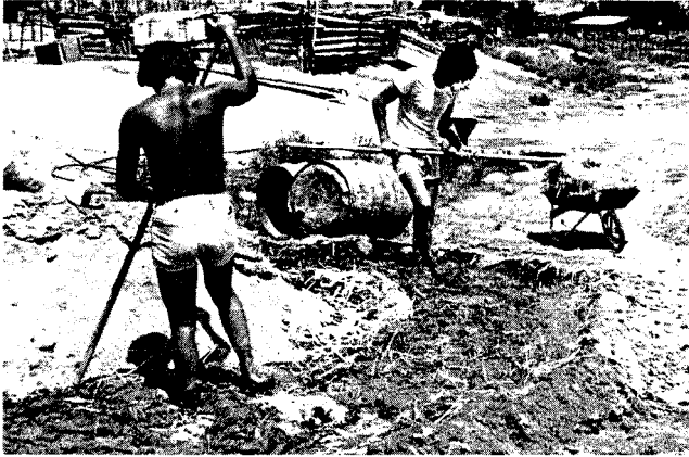
FIGURE 60-FOOT-TREADING STRAW INTO ADOBE IN MUDPIT; Roman Valdez and James Lujan adobe operation, Nambe.
