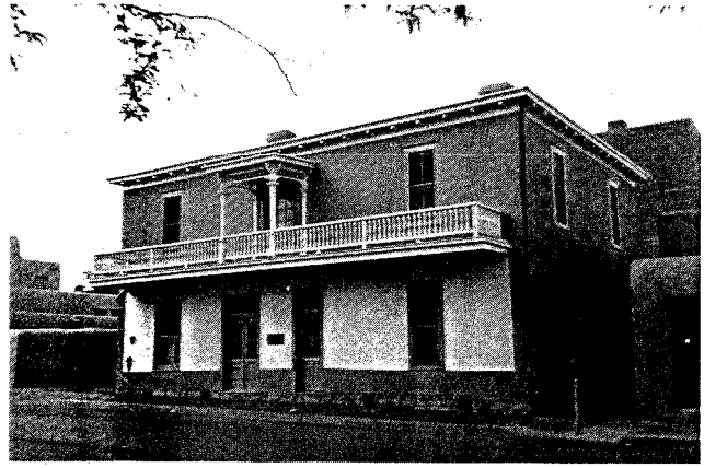
FIGURE 10—FELIPE S. DELGADO BUILDING IN SANTA FE, REPRESENTATIVE OF TERRITORIAL STYLE ARCHITECTURE.
