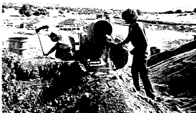
A--SHOVELING ADOBE SOIL INTO TRACTOR-MOUNTED CEMENT MIXER
