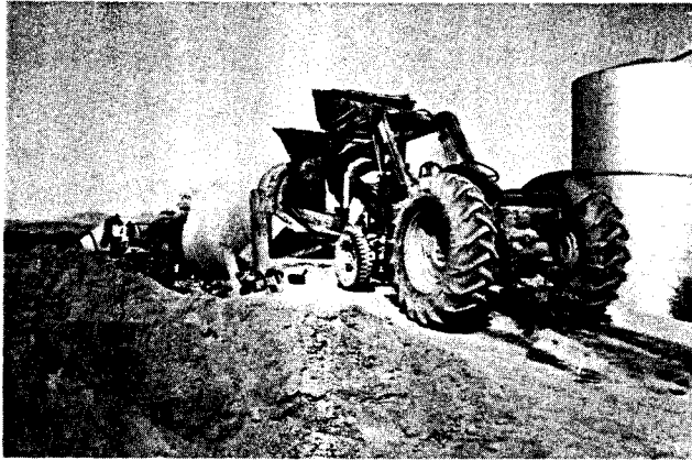
A—FRONT-END LOADER PLACING ADOBE SOIL INTO HOPPER OF CEMENT MIXER.
