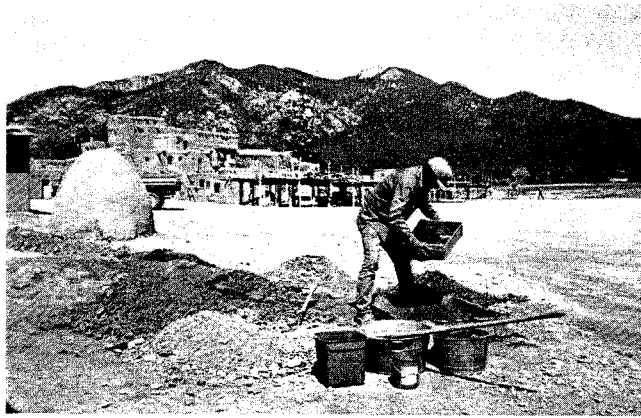
FIGURE 29—SCREENING ADOBE SOIL FOR REPLASTERING HOMES IN TAOS PUEBLO.
