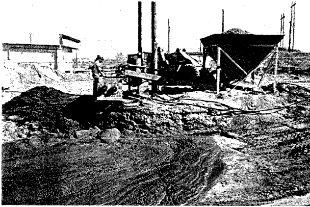
D- ADOBE MUD IS DUMPED INTO LARGE MUDPIT
