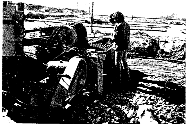
B-ADOBE MATERIAL IS CONVEYED TO SCREEN THAT COVERS PART OF PUG-MILL TROUGH WHERE LARGE GRAVEL IS REMOVED.
