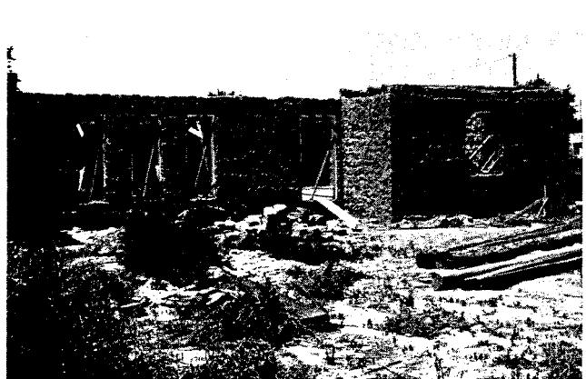
E TERRÓN HOUSE UNDER CONSTRUCTION DURING SUMMER OF 1980.
