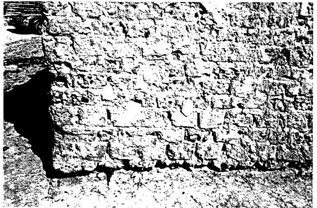
FIGURE 33—UNDERCUTTING OF ADOBES AT GRADE LEVEL; note size of gravel in adobe bricks.
