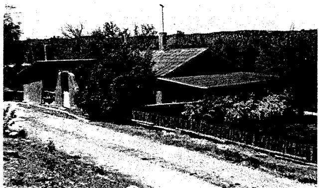
FIGURE 34—OLD TIN-ROOFED ADOBE HOUSE BELONGING TO AUTHOR. LOCATED IN TESUQUE. Roof was added to protect original adobe long-house structure and to cover dirt-roof area.
