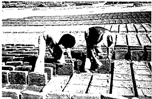
I-AFTER DRYING FOR 2 OR 3 DAYS, ADOBES ARE TURNED ON EDGE AND TRIMMED OF EXCESS MATERIAL.
