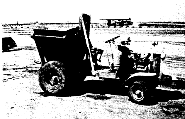
D—ONE-TON MUD BUGGY DEVELOPED BY HANS SUMPFF COMPANY FOR CARRYING MIXED ADOBE MUD FROM PUGMILL TO ADOBE LAYER.
