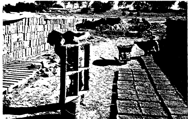
D - FORM IS THEN WASHED AND REPLACED TO AWAIT NEXT POURING OF ADOBE MUD.
