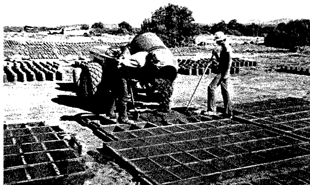
C-TRACTOR MIXER DUMPS ADOBE MUD INTO WOODEN MOLDING FORMS
