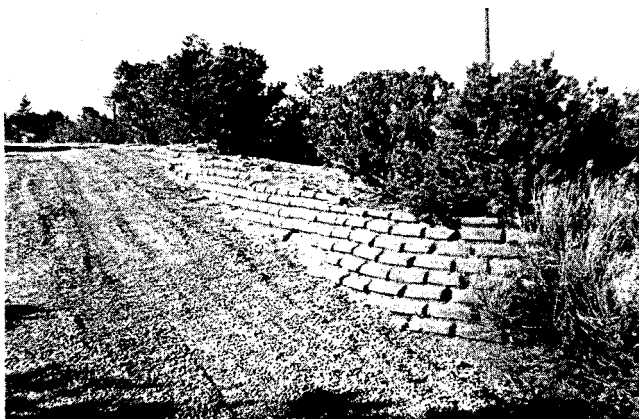
FIGURE 44-DRIVEWAY RETAINING WALL BUILT OF STABILIZED ADOBE BRICKS. SANTA FE.
