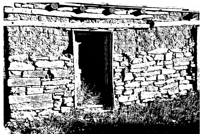
FIGURE 28-COMBINATION OF FIELD STONE AND ADOBE BRICKS. SAN JOSE.
