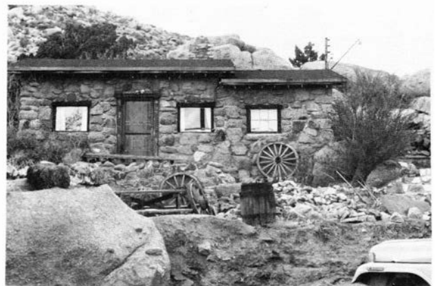
FIGURE 81—DWELLING IN TIJERAS CANYON SOLIDLY BUILT OF SANDIA GRANITE.
