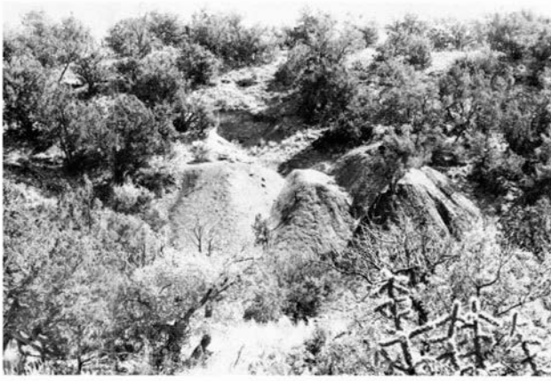
FIGURE 90—SECTION 1 MINE IN TIJERAS BASIN. ERODED DUMP AND PARTLY CAVED PORTAL TO INCLINE.
