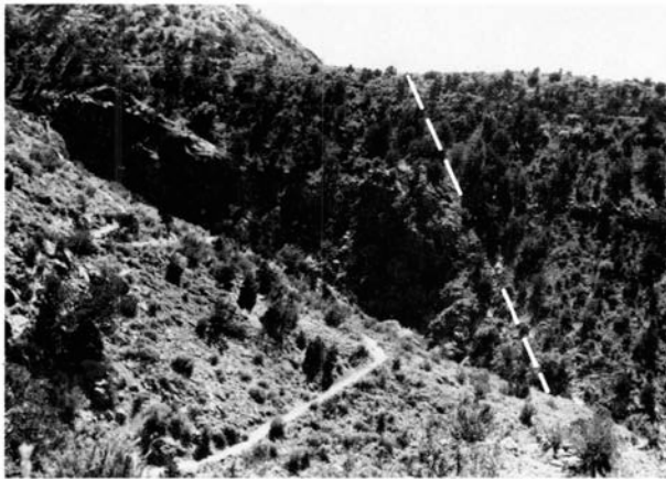
FIGURE 56—FAULTED SANDIA GRANITE IN CANYON SIDE NEAR BOTTOM OF LA LUZ TRAIL. THIS FAULT FORMS THE BASE OF THE PROMINENT TRIANGULAR FAULT-FACETED SPURS NORTH AND SOUTH OF LA CUEVA CANYON.
