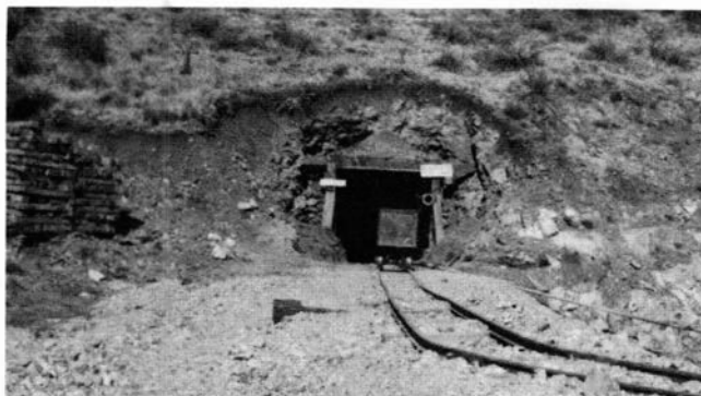
PHOTO 2—CLUM MINE, GRANT COUNTY; LETRADO ADIT CROSSCUT (portal located on north slope of hill about 165 ft below outcrop of main Clum vein).
