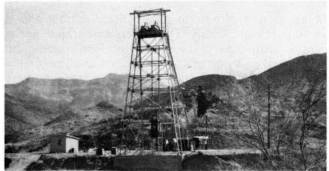
PHOTO 7—LYDA K MINE, SIERRA COUNTY; NEW HEADFRAME ON OLD NO. 1 SHAFT AND OLD WORKINGS ON LYDA K VEIN (view to northeast; Caballo Mountains in background).
