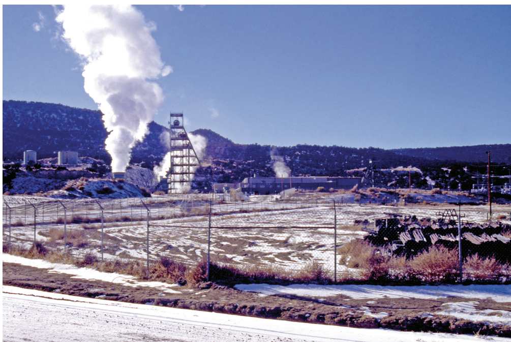
Steam rising from the head frame at the Mt. Taylor mine (NMC10027), Ambrosia Lake subdistrict, Grants uranium district. The Mt. Taylor mine is 3,300 ft deep. Photo by Virginia T. McLemore.
