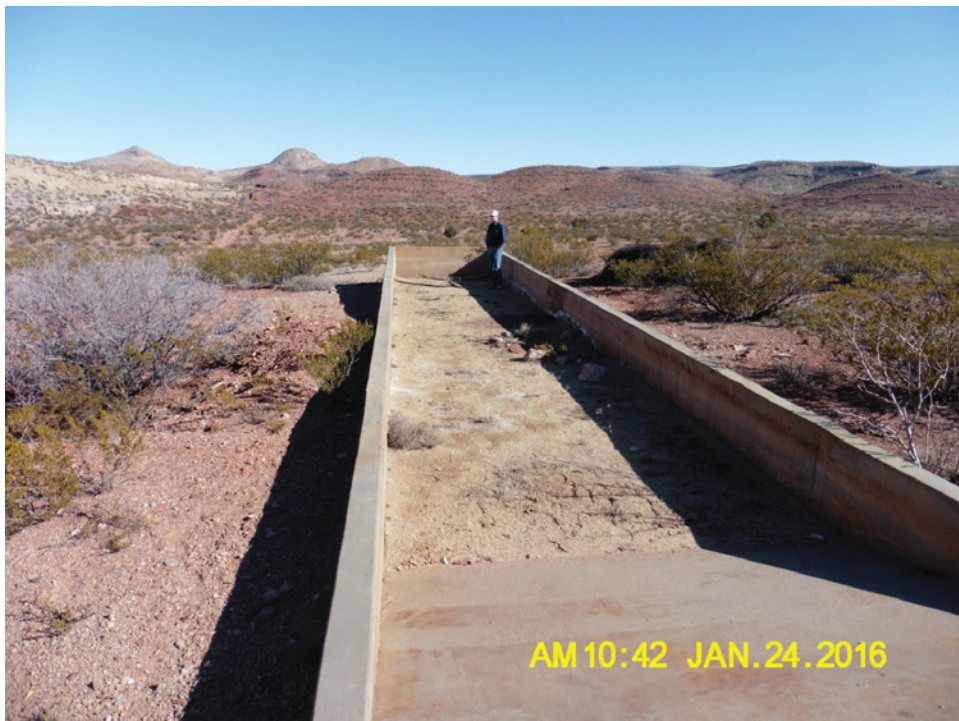
Figure 92. Leach tanks at Minas del Chupadera, looking east. Photo by V.T. McLemore, 1/24/2016
