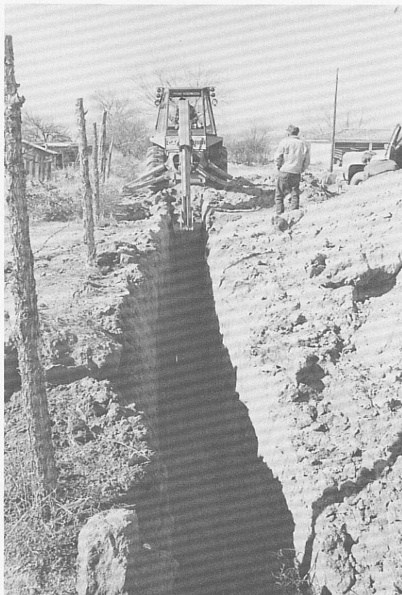
PHOTOGRAPH 4—Exploratory trench that was used for visual examination and sampling of near-surface soils.
