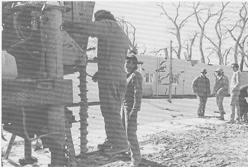
PHOTOGRAPH 3—Equipment used for drilling geotechnical wells and obtaining laboratory samples. Note damaged house in background.
