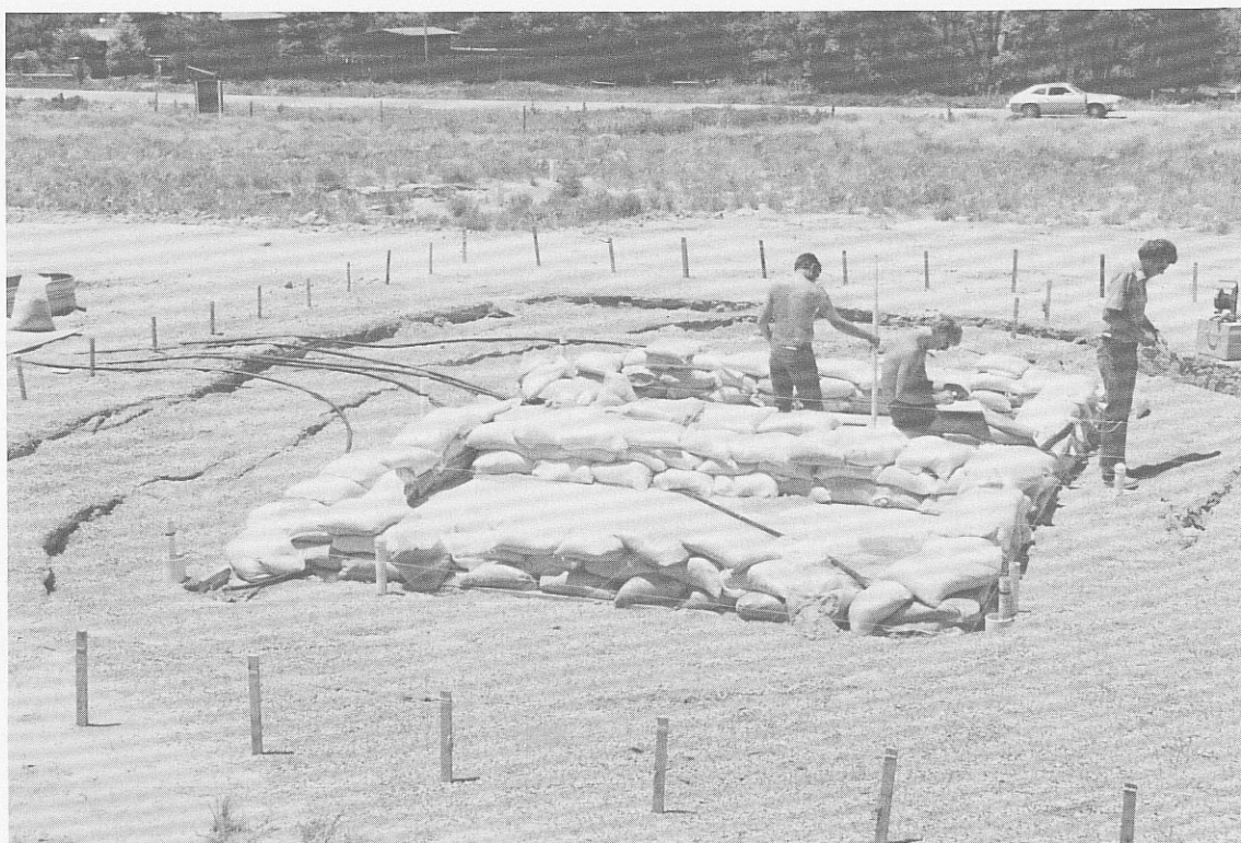
PHOTOGRAPH 10—Geotechnical ground stabilization study area 4 showing near-to-maximum surface settlement and ground cracks on June 10, 1985 (view to the west).
